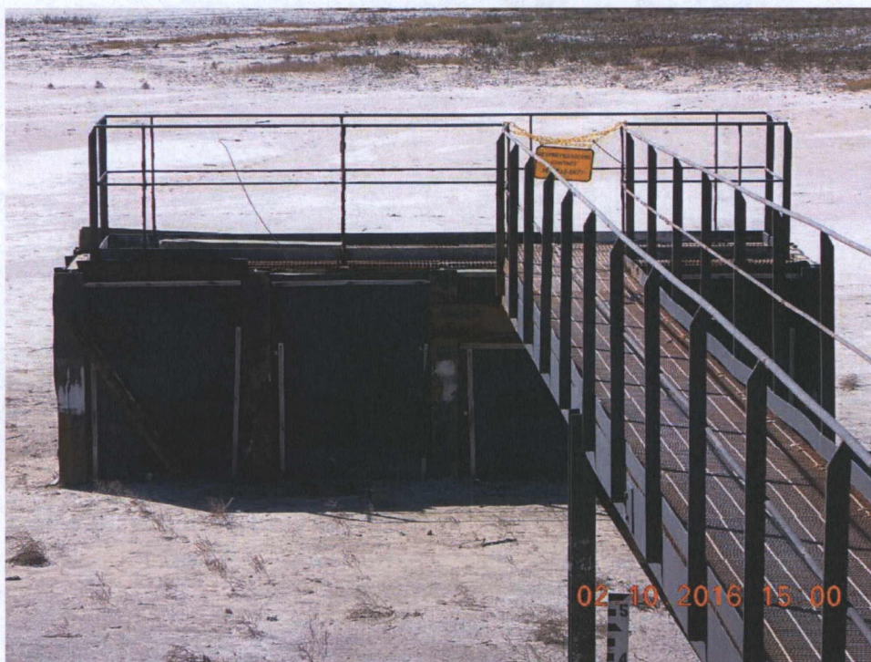
Figure 6 - North Decant Structure
