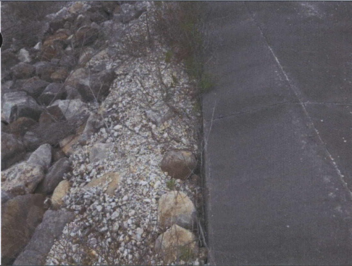
31 – Emergency Spillway, viewing minor washout along edge
