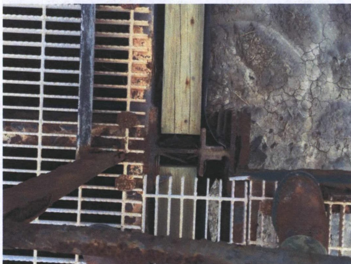
North Decant Structure Corrosion
