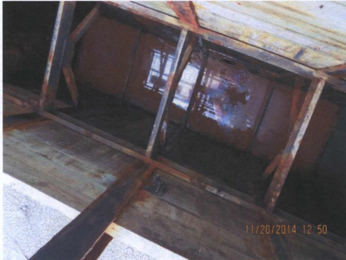
South Decant Structure Corrosion (inside)
