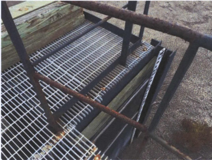
South Decant Structure Corrosion
