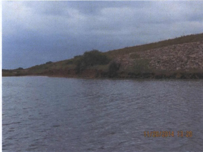
NE CDF External Slope, Cut Near Toe from Dredge Operations
