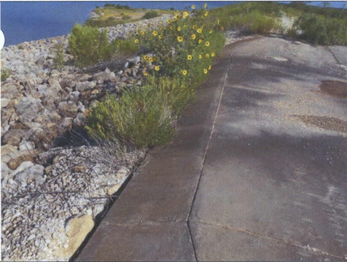
31 – Emergency Spillway, viewing minor washout along edge
