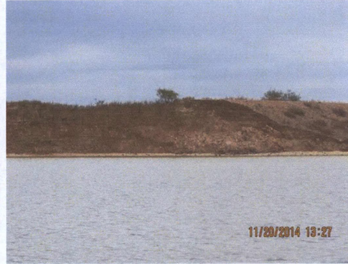
South CCND Dike Erosion (exterior)
