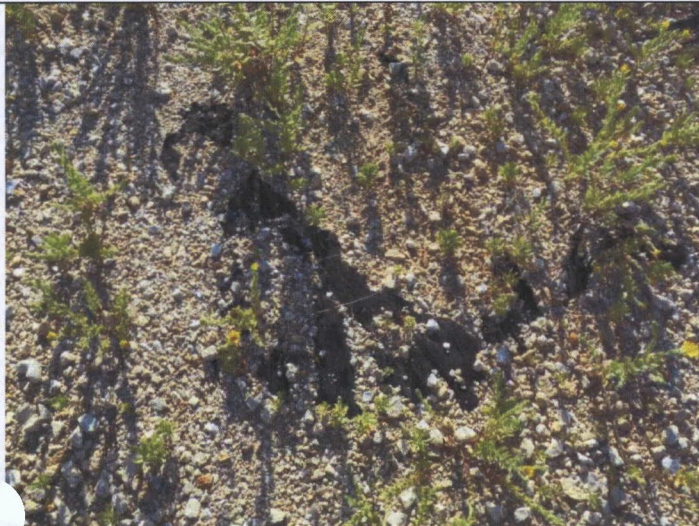
5 – Northeast Conner Outer Dike, viewing moderate exposure of the geomembrane
