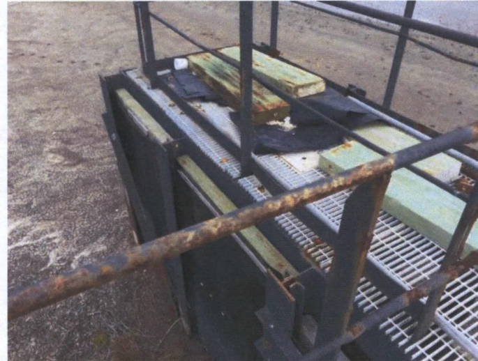
South Decant Structure Corrosion
