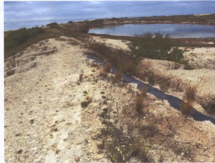
CCND Dike Erosion at Water Stop (East Side, Facing South)
