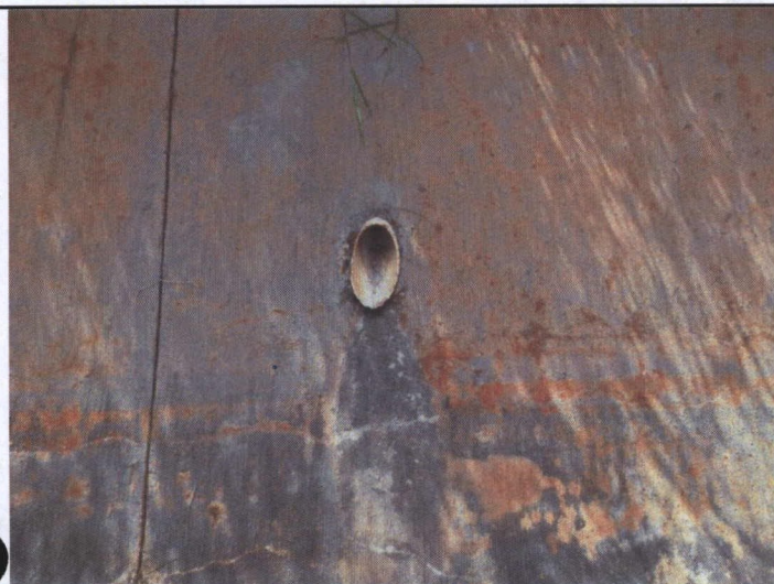
17 – View of minor erosion under inlet pipe
