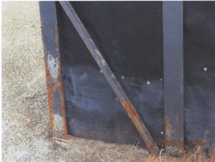
South Decant Structure Corrosion
