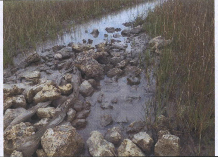
16 - View of minor movement of rip rap at the end of the drainage channel
