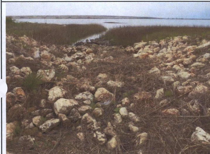
9 - View of rip rap at the end of the drainage channel
