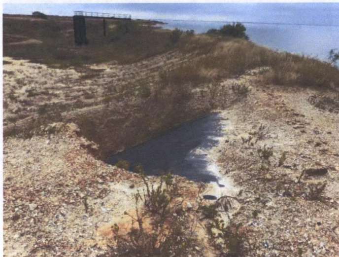
CCND Dike Erosion at Water Stop (West Side, Facing South)
