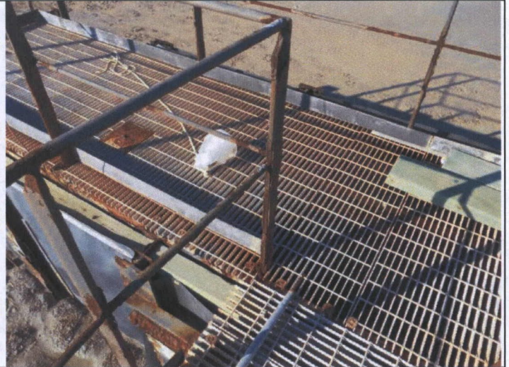
34 – North Decant Structure, viewing rust on structural members
