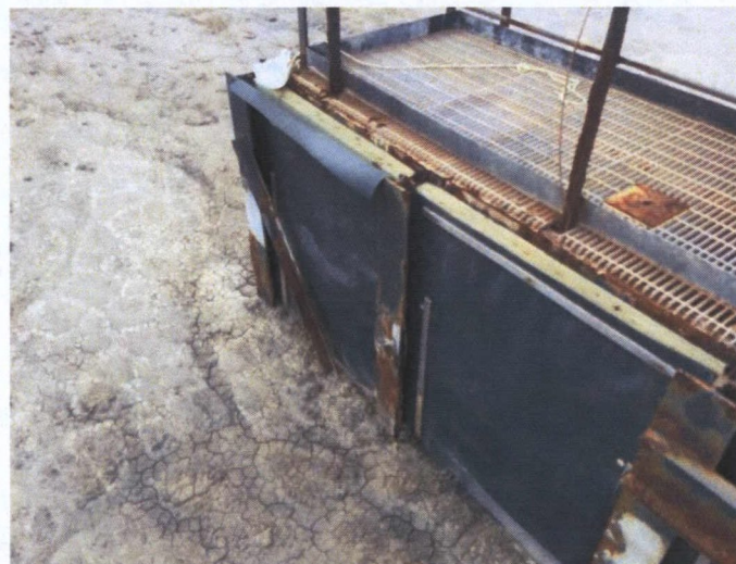
North Decant Structure Corrosion
