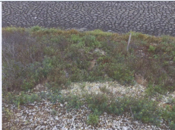
4 – North Inner Dike, viewing erosion damage
