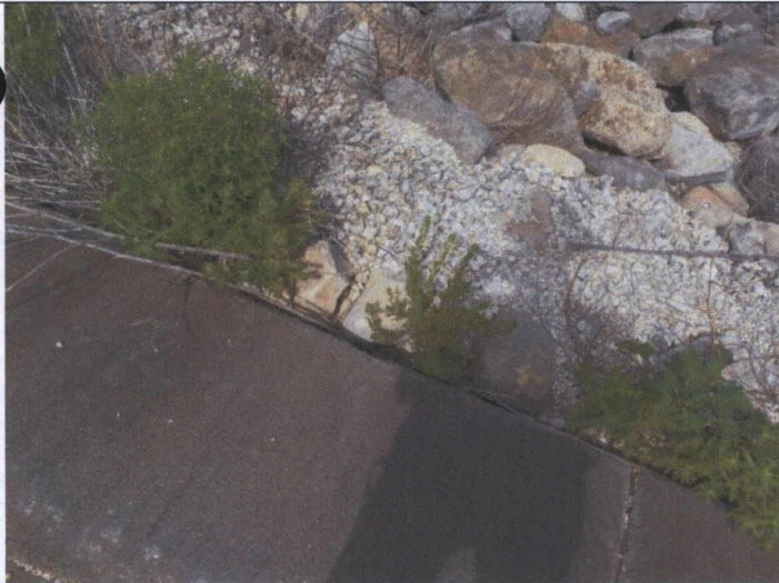
31 – Emergency Spillway, viewing minor washout along edge
