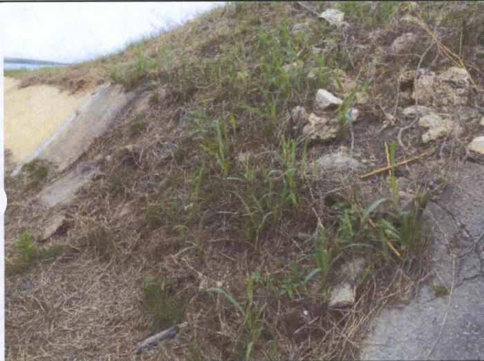
15 - View of deteriorating side slope on channel
