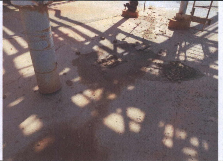
2 - Cap, storm sewer drain at R-301
