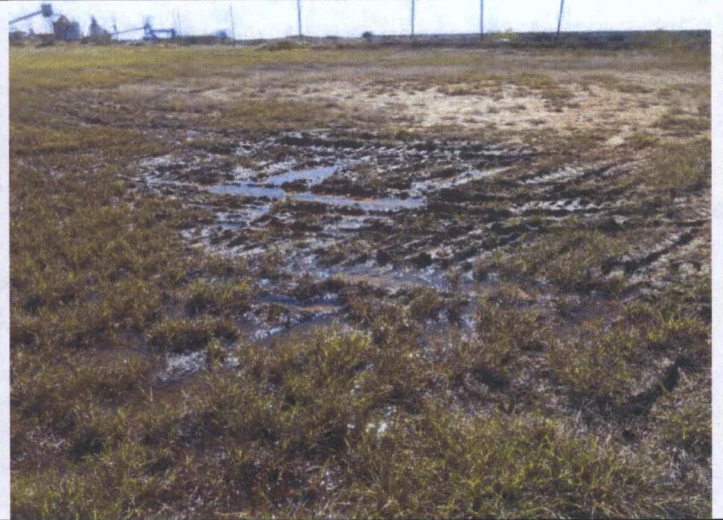
16 - View of rutting on the O/W Separator Cap
