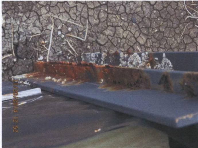
South Decant Structure Corrosion
