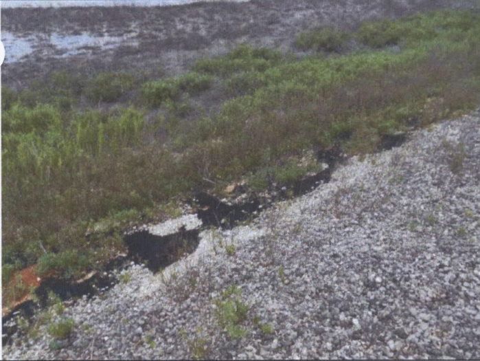
19 – South Dike, viewing exposed geomembrane
