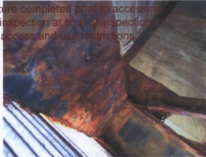
North Decant Structure Corrosion (inside, near grate surface)
