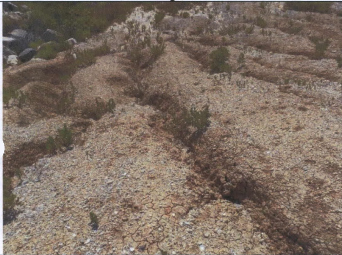
33 – East CPA Outer Dike, viewing erosion
