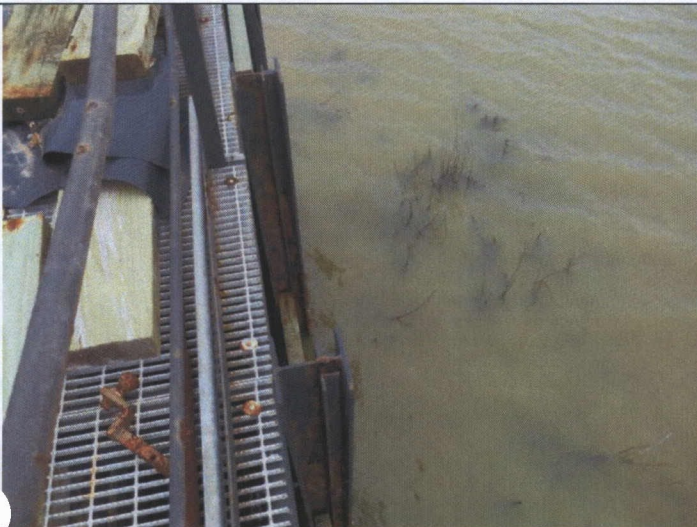
36 – South Decant Structure, viewing rust on structural members
