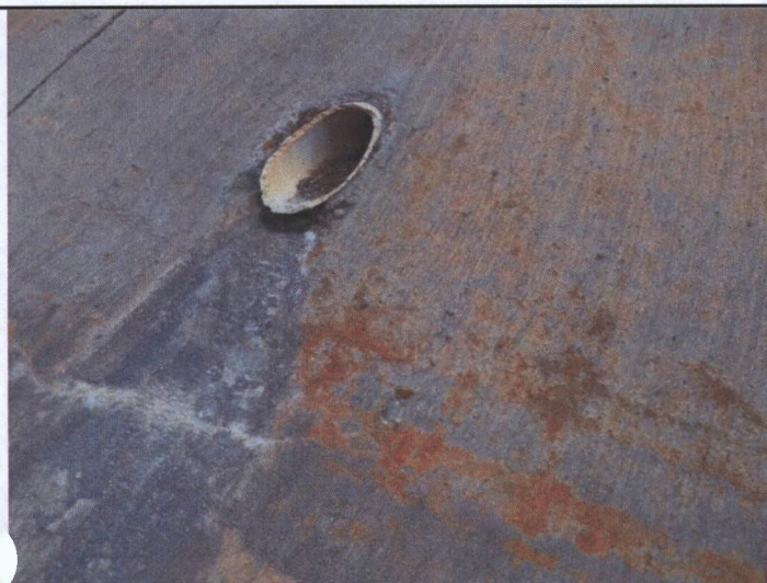
17 – View of minor erosion under inlet pipe
