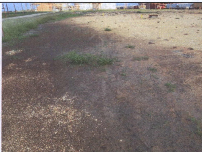
12 – Cap, Ruts from herbicide treatment and soil building up on edge of cap
