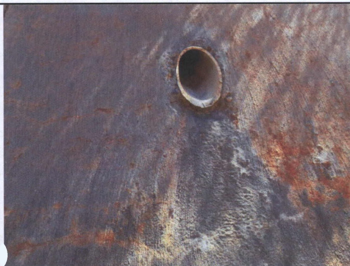
17 – View of minor erosion under inlet pipe
