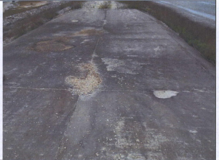
30 – Emergency Spillway, viewing minor deterioration of the concrete
