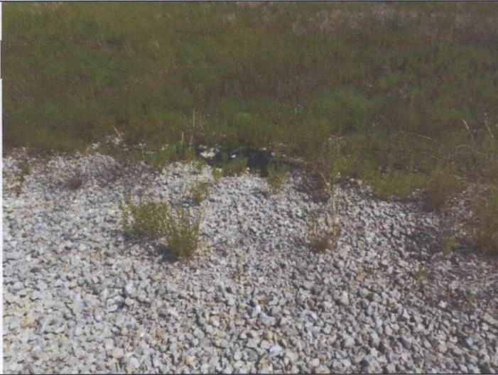
19 – South Dike, viewing exposed geomembrane
