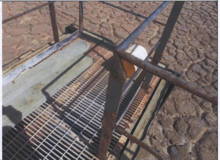
34 – North Decant Structure, viewing rust on structural members
