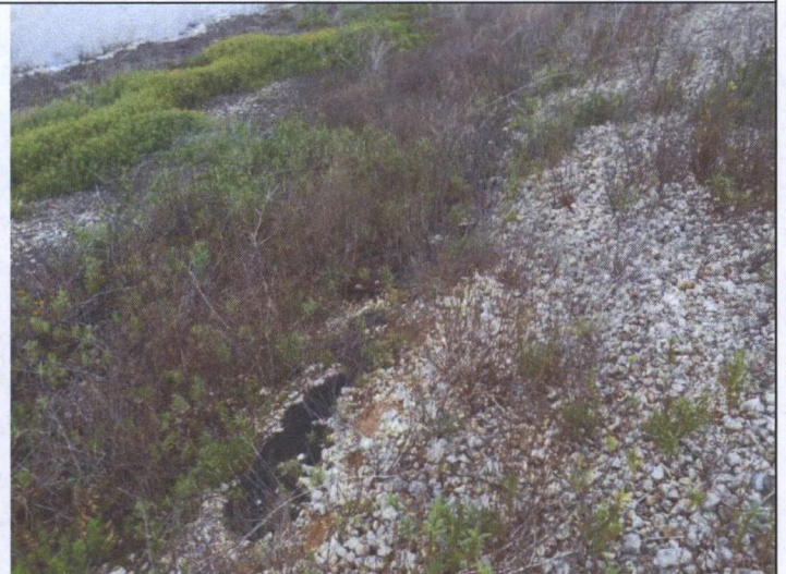
24 – West Inner Dike, viewing exposed geomembrane
