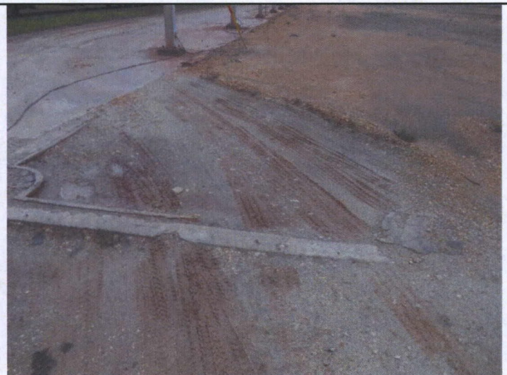
12 – Cap, Ruts on Northeast corner
