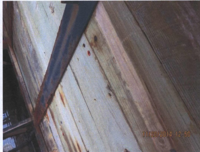
South Decant Structure Corrosion (inside)
