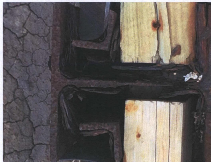
North Decant Structure Corrosion
