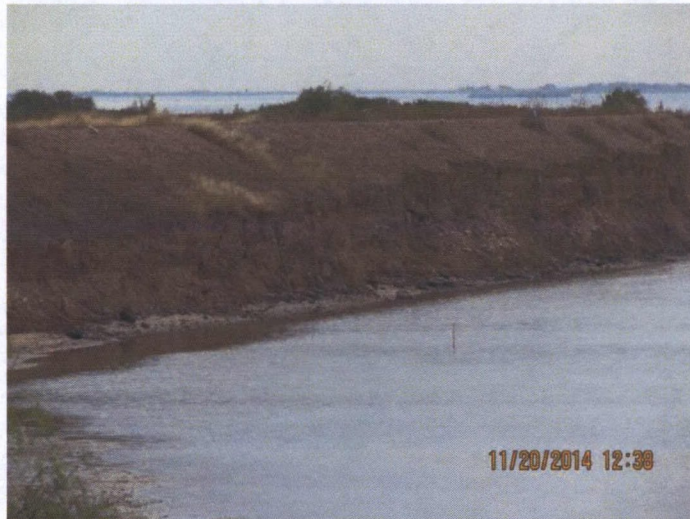
NE CDF External Slope, Cut Near Toe from Dredge Operations
