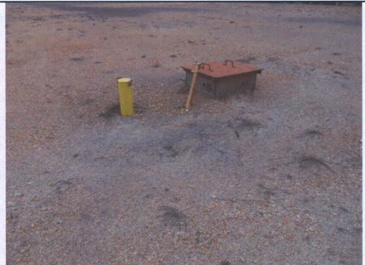
10 – Cap, Not in service extraction well
