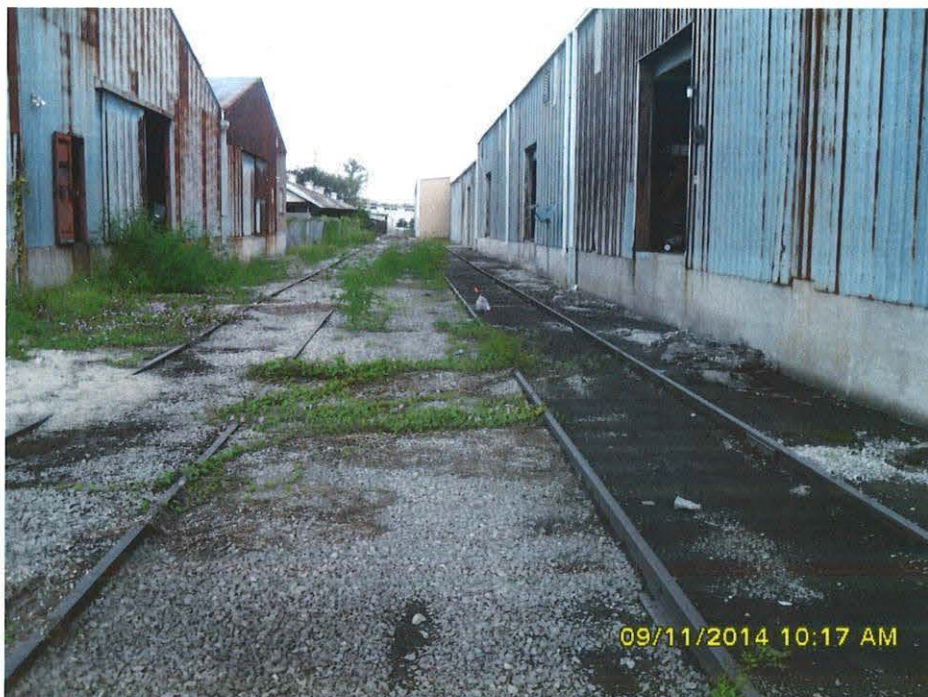
View Grid AD-010, which was determined to contain Libby Amphibole Asbestos.
