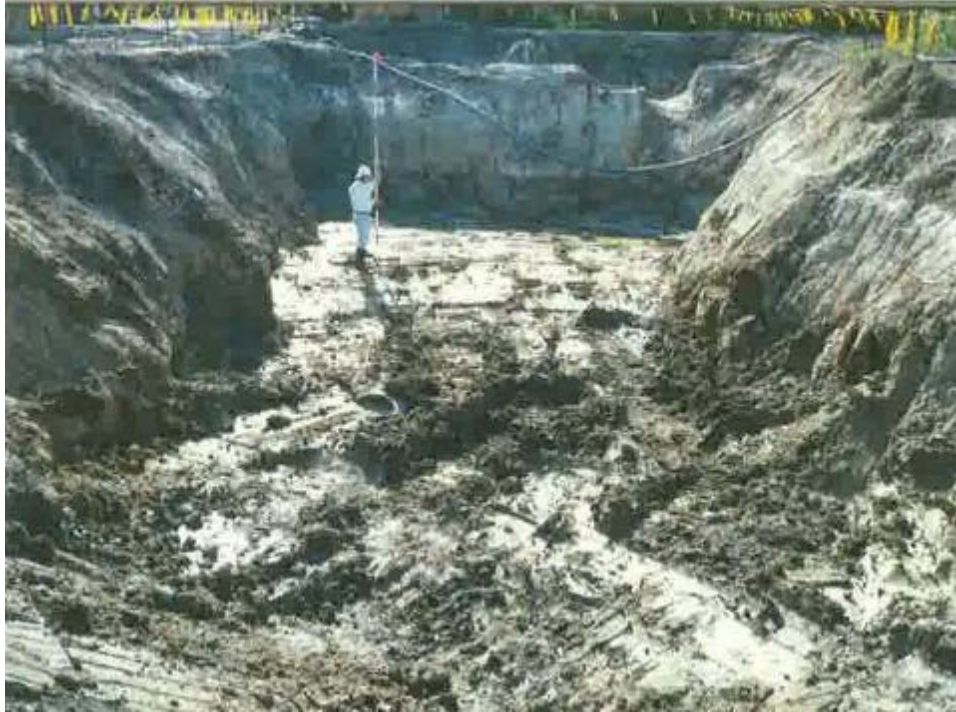
Survey of excavated pond bottom to support excavation volume calculation
