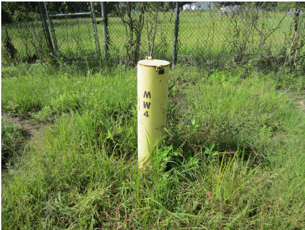
Monitoring well MW-04 located in the southwest corner of the former Pond Area
