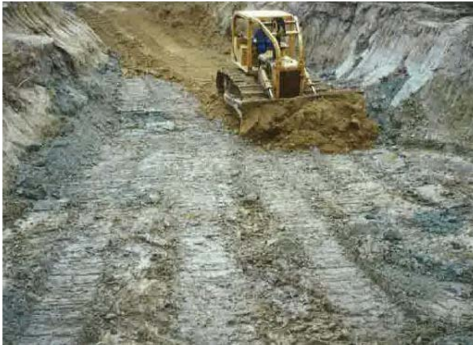
Pond bottom receiving first layer of backfill
