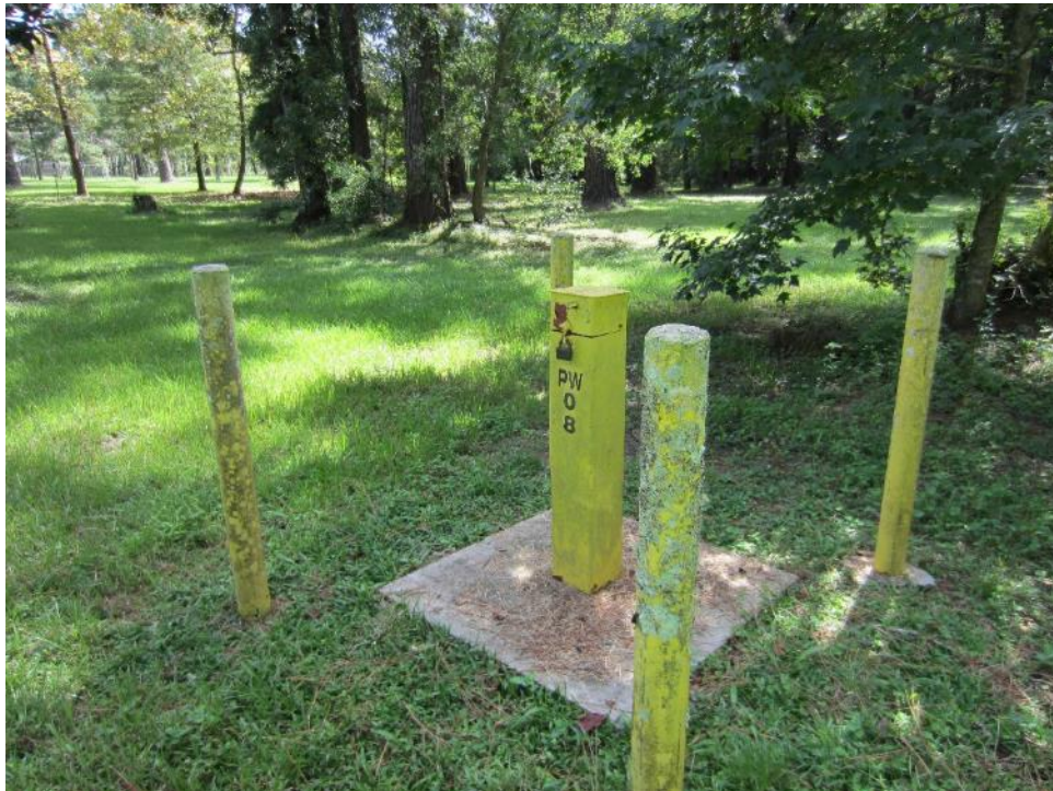
Monitoring well PW-08 located north of Stand G
