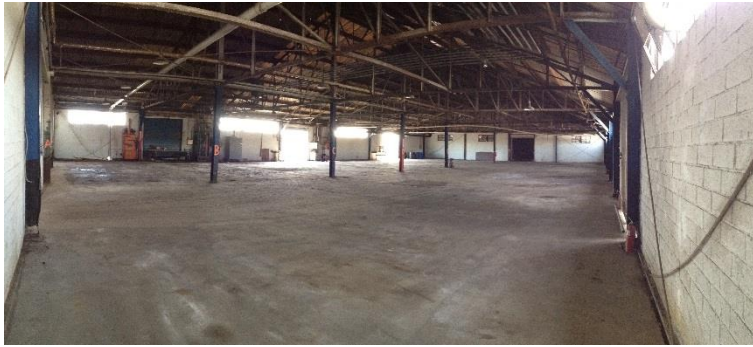
400 N. Richey Warehouse after Removal/Disposal (Jan 2015)
