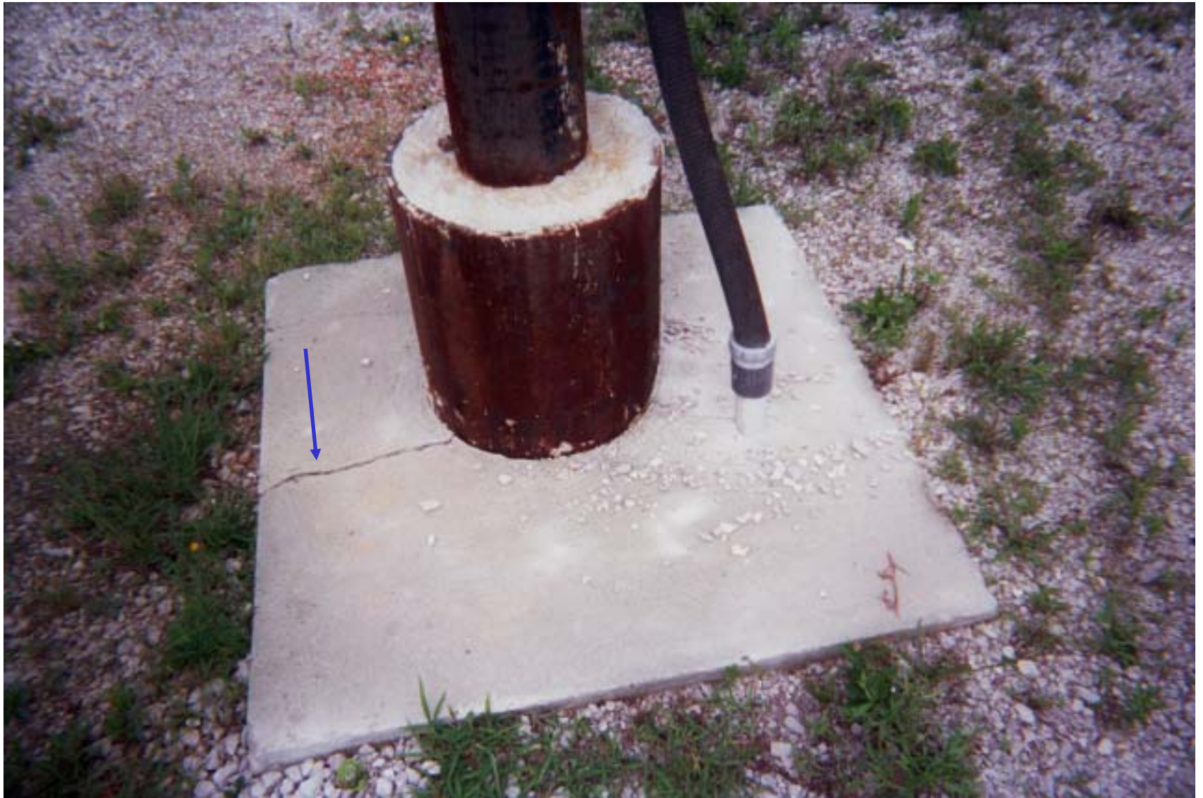
Photo 52: View of well pad for Quapaw #5 MW. Well pad is cracked (blue arrow).
