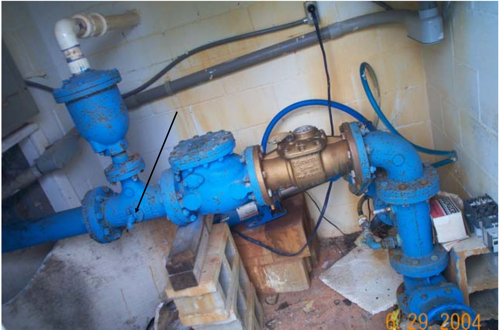
Photo 4: View inside the well house of the Picher #5 MW. Faucet used for sample collection is shown at black arrow.
