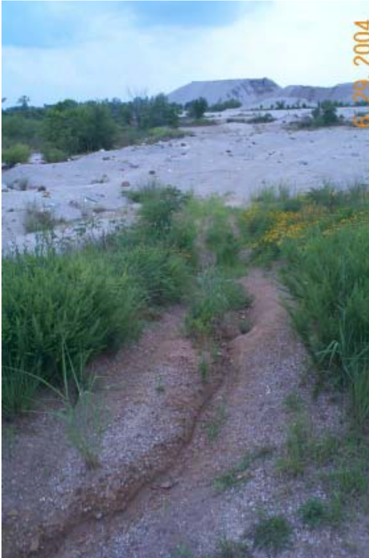
Photo 12: View along the south side of the diversion dike at the Admiralty Mine site.
