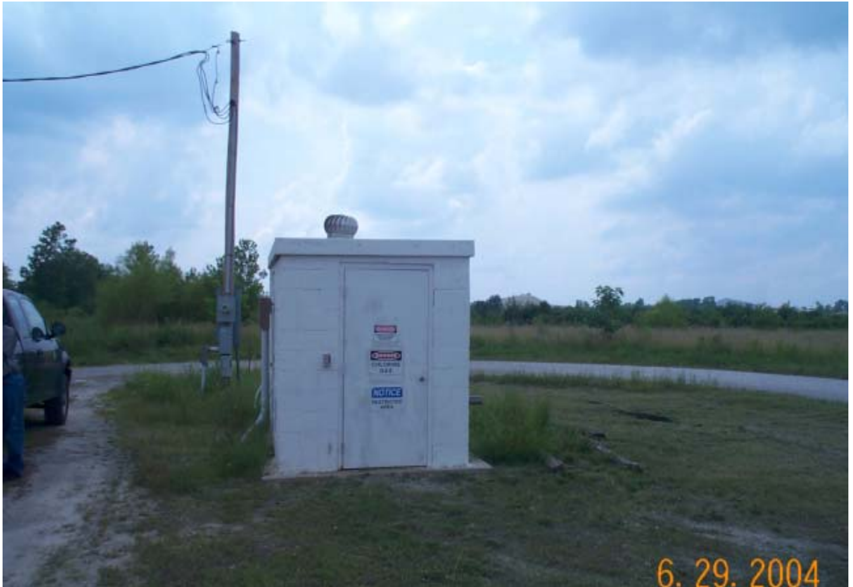
Photo 3: View of the Picher #5 MW. The City of Picher has erected a well house over the well-head and connected this well to the City water supply.
