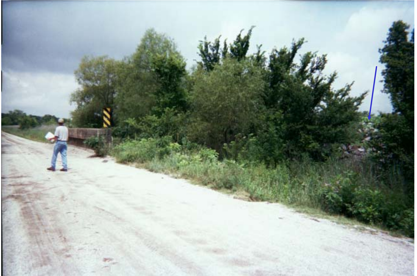
Photo 66: View of road on south side of diversion dike at Big John Mine site, located in Kansas. The backside of the diversion dike is barely visible through the trees (at blue arrow). The bridge is where the old Tar Creek channel used to flow.
