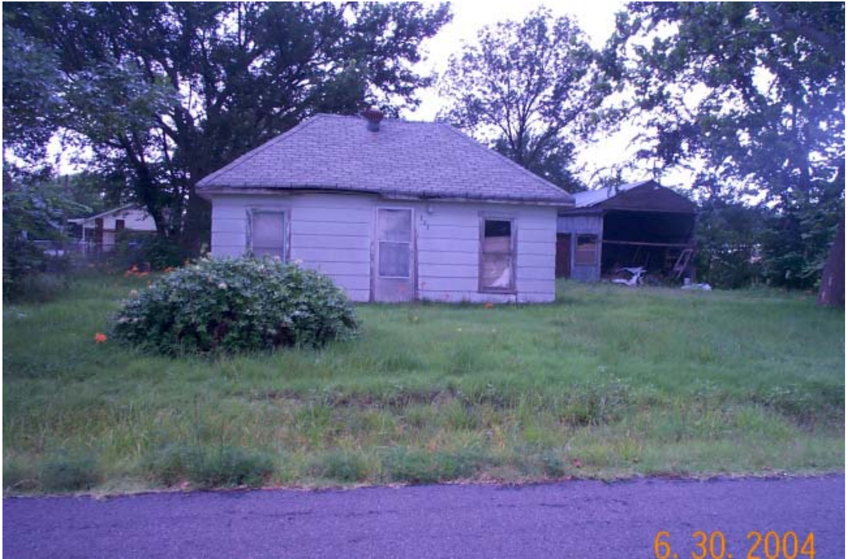
Photo 31: View of unremediated property in North Miami, Oklahoma.
