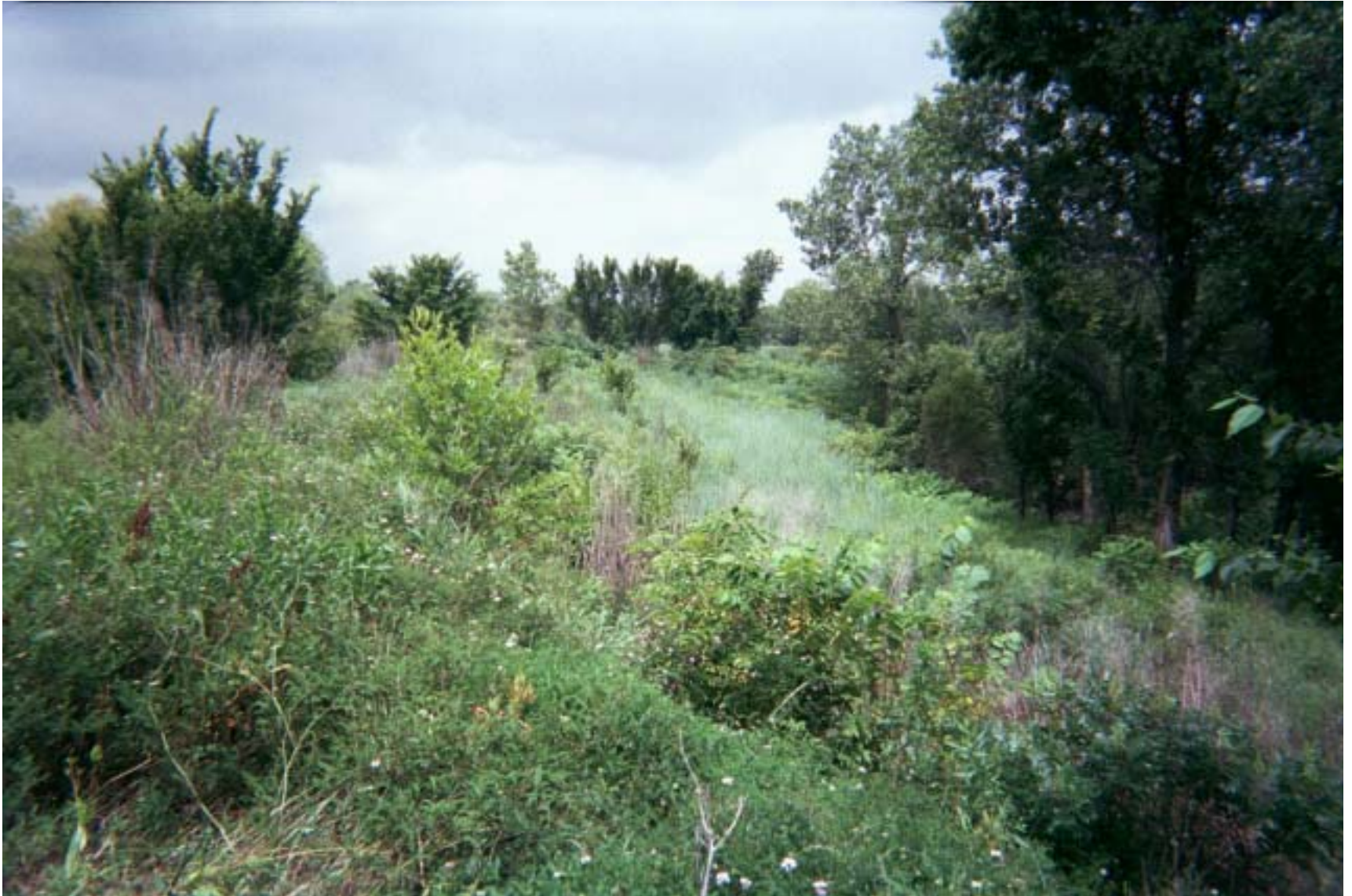
Photo 64: View of diversion dike at the Big John Mine site, located in Kansas. The subsidence feature is located to the right of this view.
