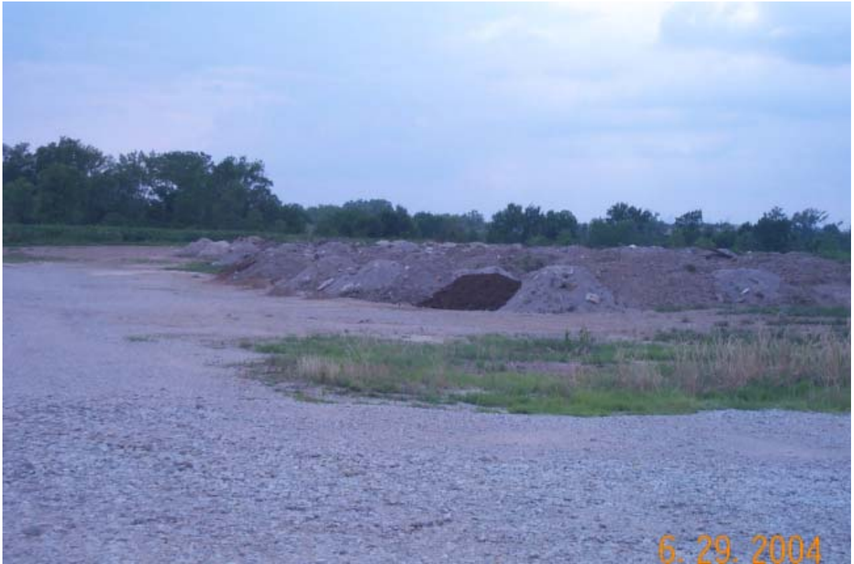
Photo 24: View of recently deposited soil at repository on E40 Road. Lead contaminated soil from residential yards is used at the repository to fill in an old mill pond.
