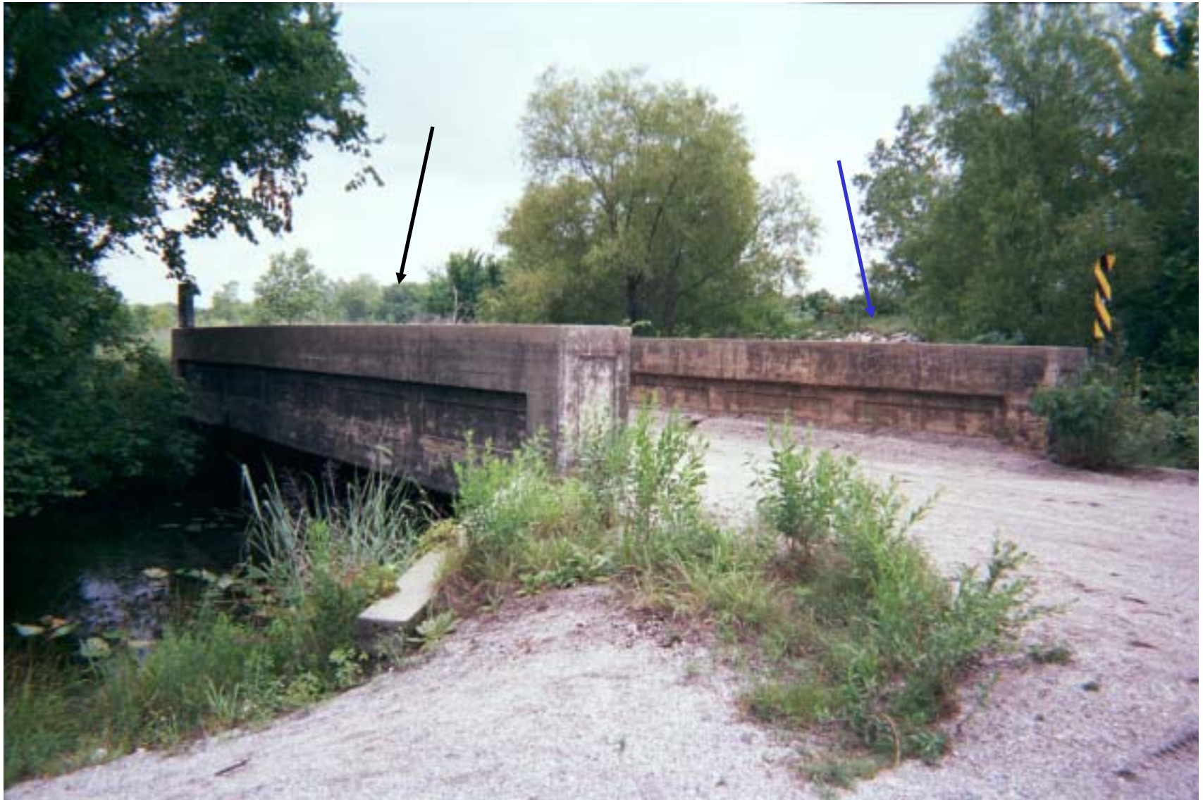
Photo 67: View of the bridge over the old Tar Creek channel at the Big John Mine site, located in Kansas (facing northwest). The backside of the diversion dike is barely visible above the bridge (at the blue arrow). Tar Creek has been diverted away from this location. The new channel is located in the trees in the background (at black arrow).
