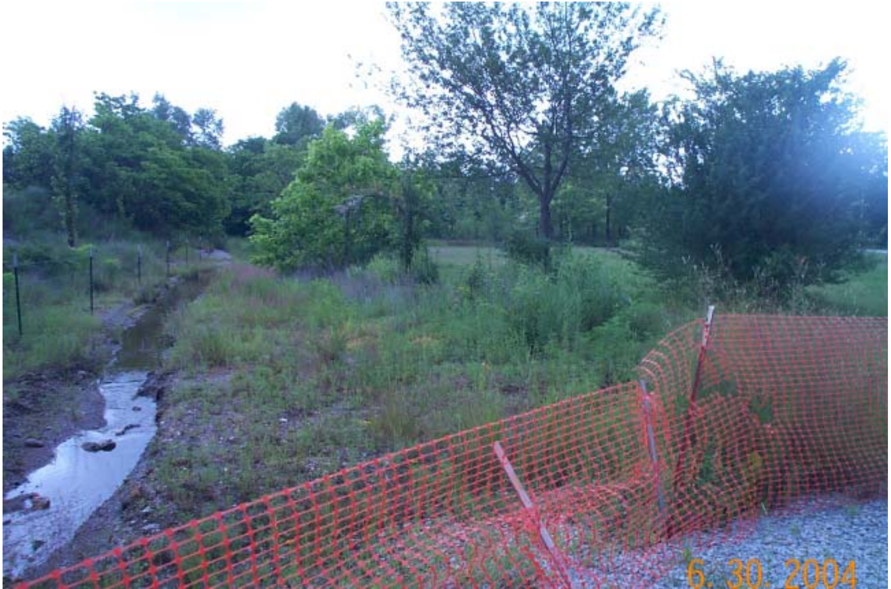
Photo 39: View of property under construction in Cardin, Oklahoma. There were still a few remaining items to complete on this property at the time of the site inspection.
