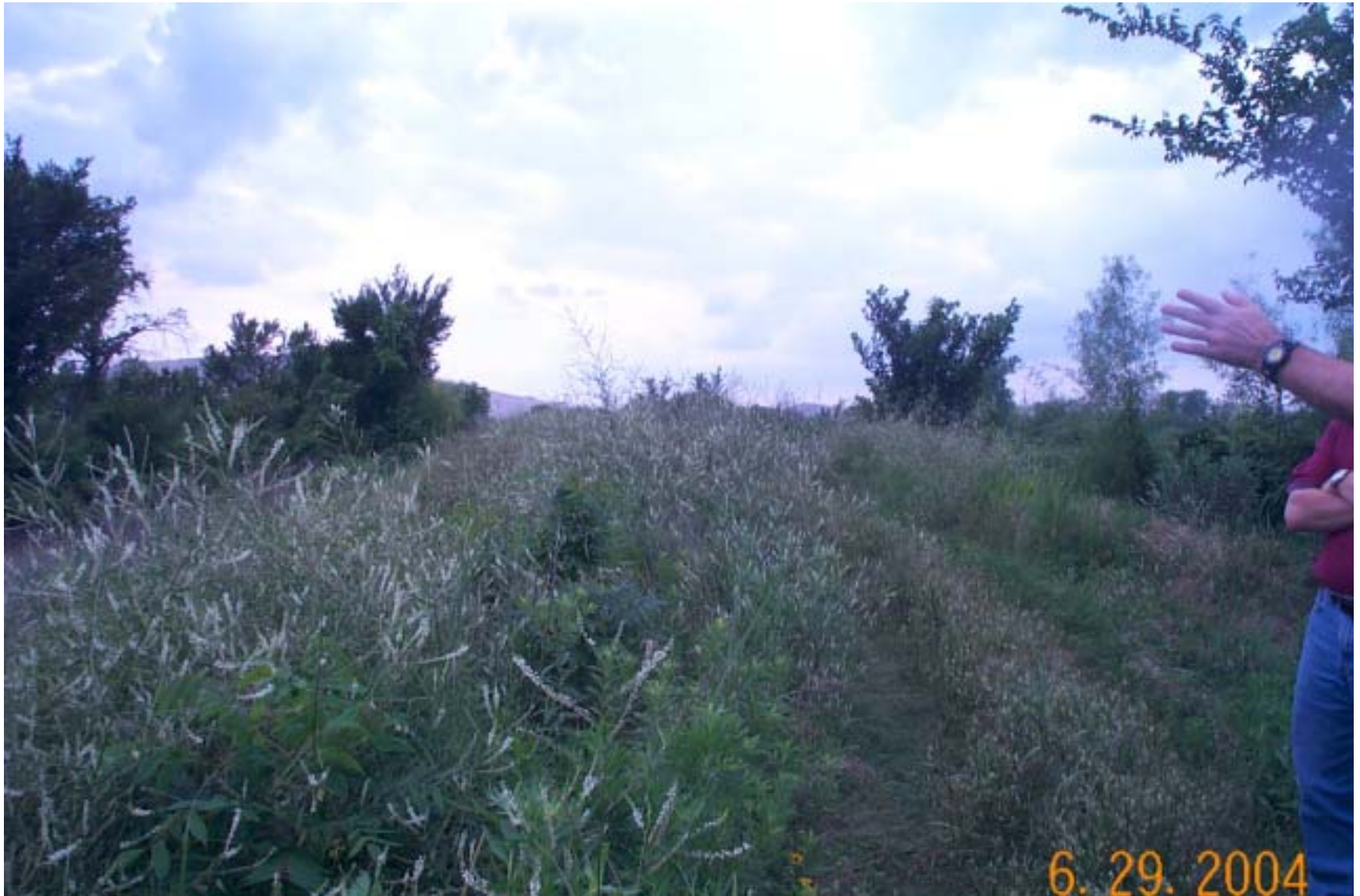
Photo 6: View of vegetative growth on top of the dike at the Admiralty Mine site.
