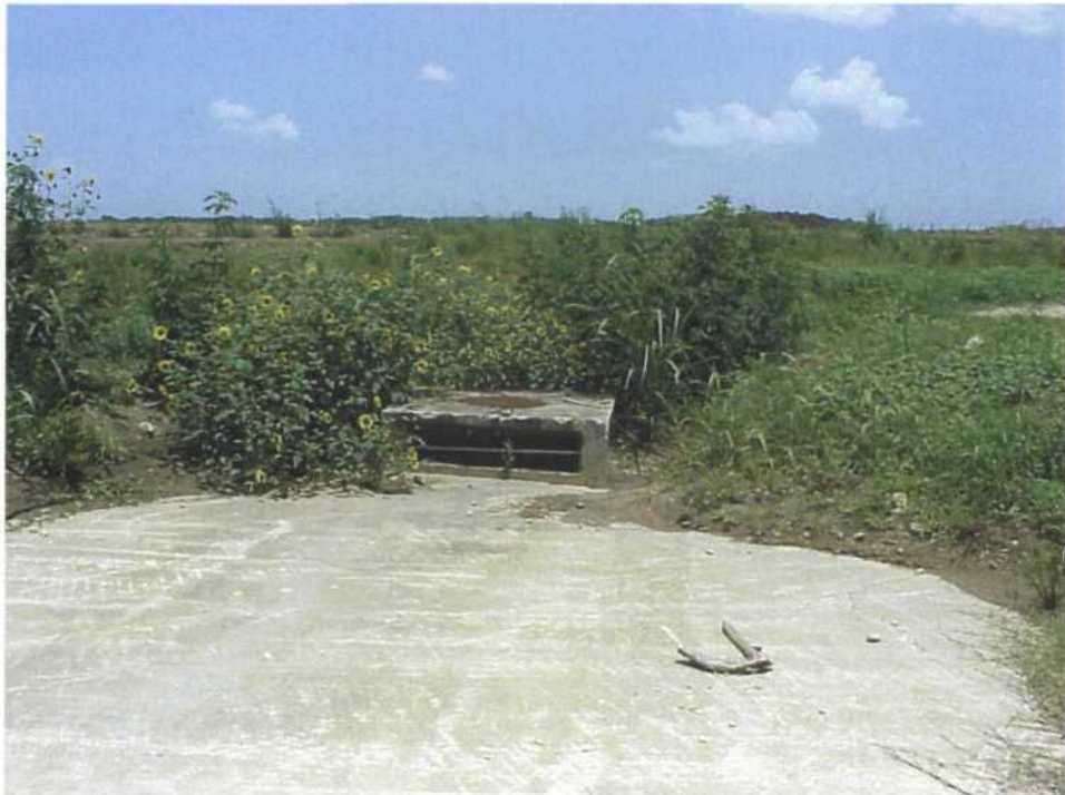
DOP-North center swale drain
