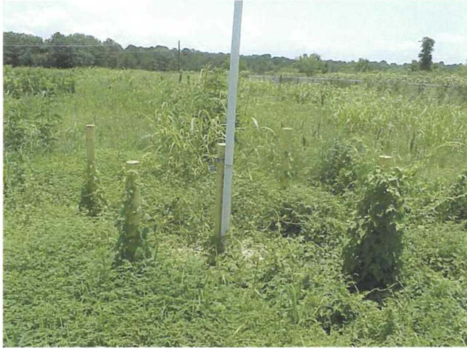
DOP-North monitor well with locator pole.
