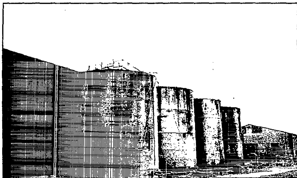
Above ground storage tanks.
