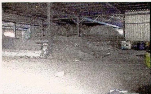
Battery Saw Building
