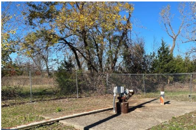
Representative monitoring well sampled quarterly by DEQ
