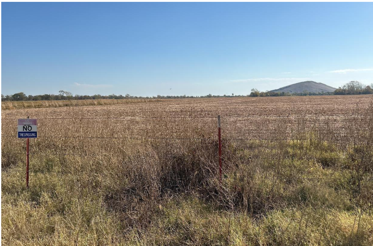
Fencing and signage posted to restrict access to a chat pile in OU4
