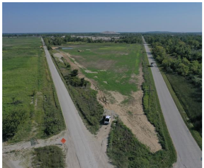
CB199 after remediation
