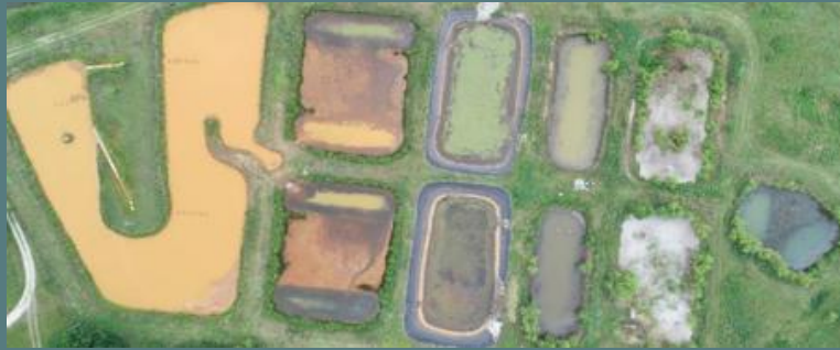
Mayer Ranch Passive Treatment System
