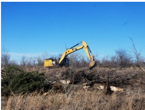
Clearing in progress at Chat Base 199
