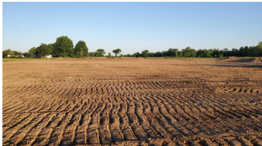
Smelter site after source removal and during final grading
