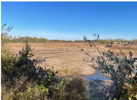
Diversion dike at Operable Unit 1
