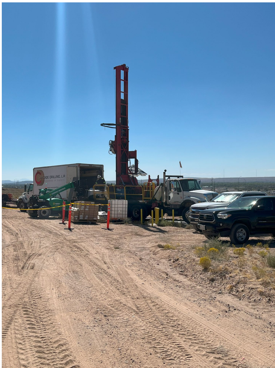
Photograph No. 6 Site: South Valley Superfund Description: OU 03, Area east of I-25; installation of additional monitoring wells.
