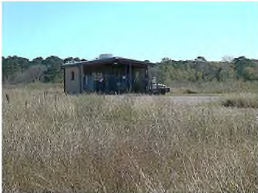
Brio North Hub C groundwater recovery system and gas collection vent (outside on the right of the building)
