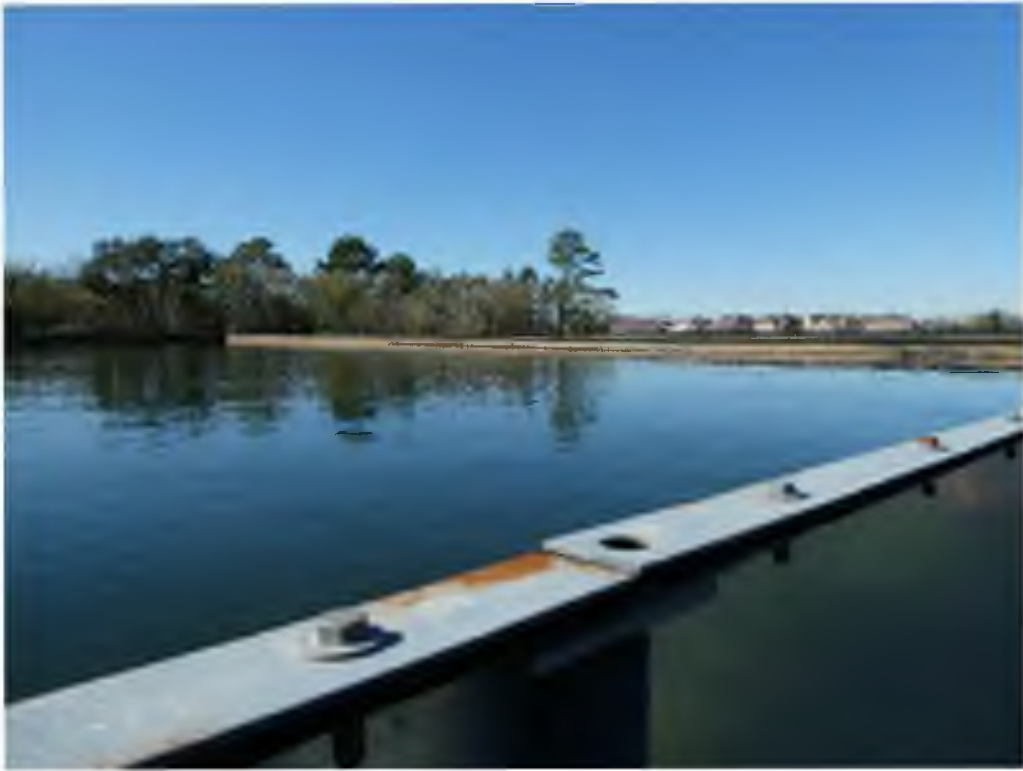
Aboveground storage pond for treated groundwater
