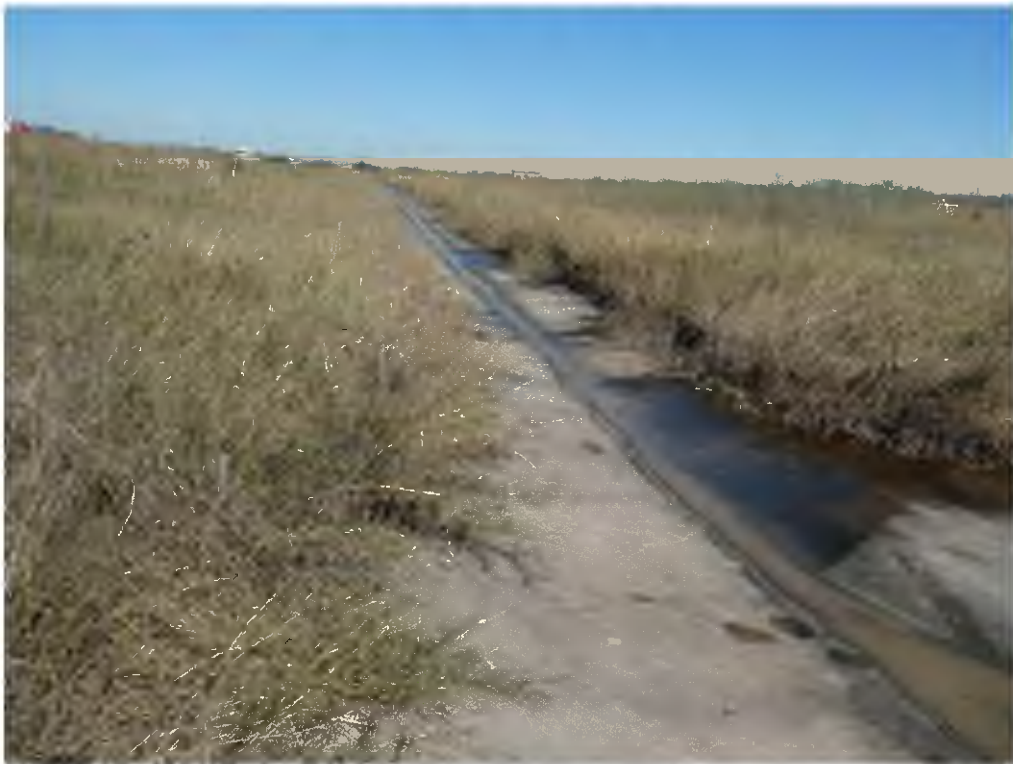
Drainage road, looking northeast from the southern boundary of Brio North
