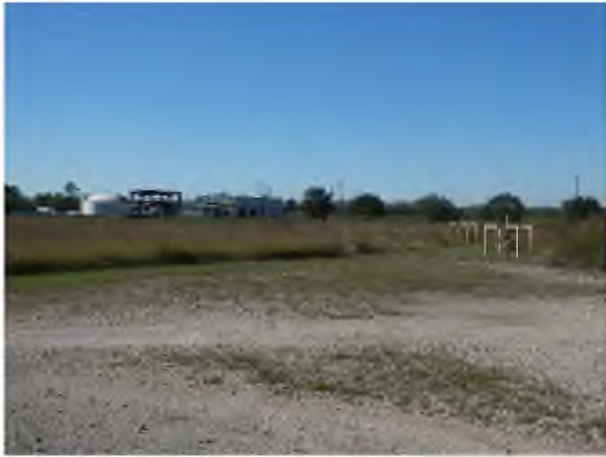
Brio North groundwater recovery wells near Hub B
