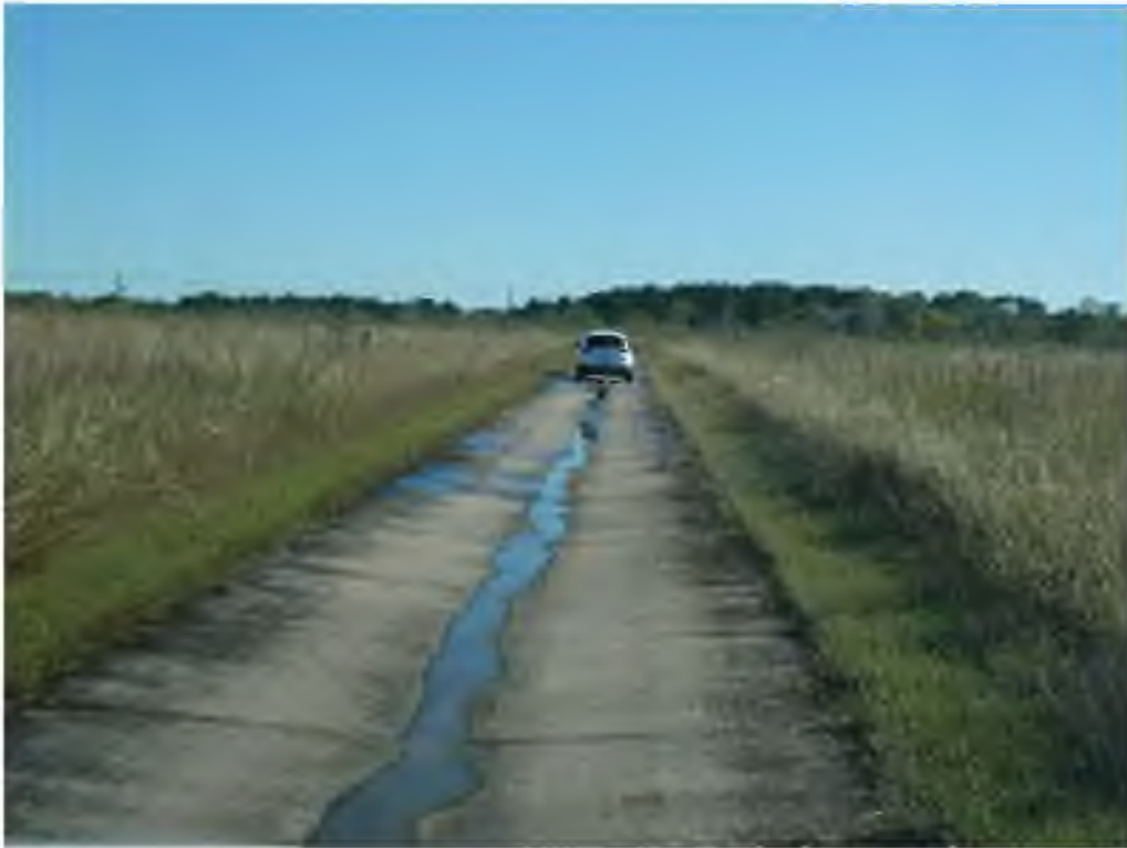
Brio North drainage road to access Hub B
