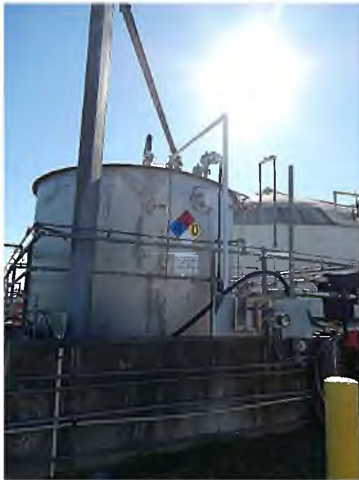
Recovered DNAPL storage tank
