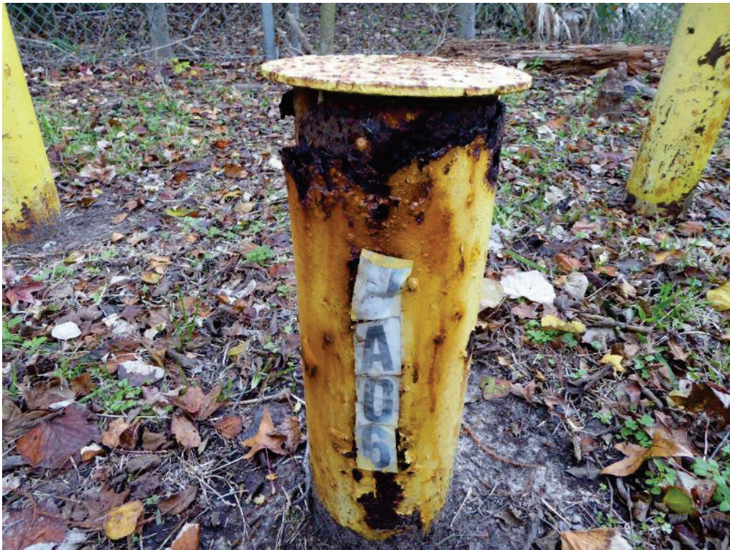
Unlocked monitoring well DA-06
