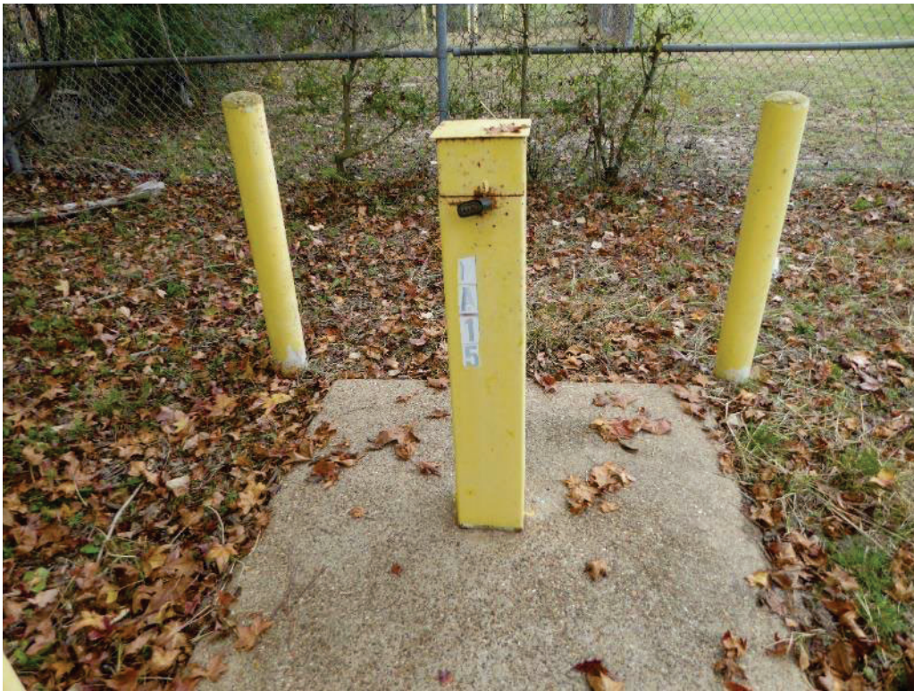
Monitoring well UA-15
