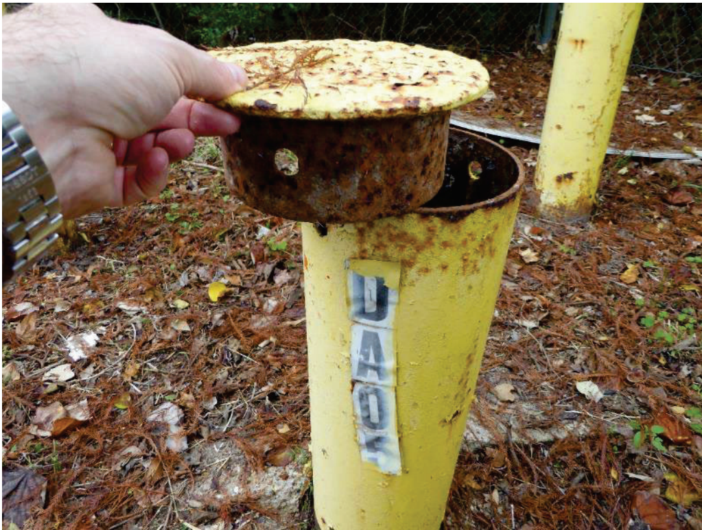
Unlocked monitoring well DA-05
