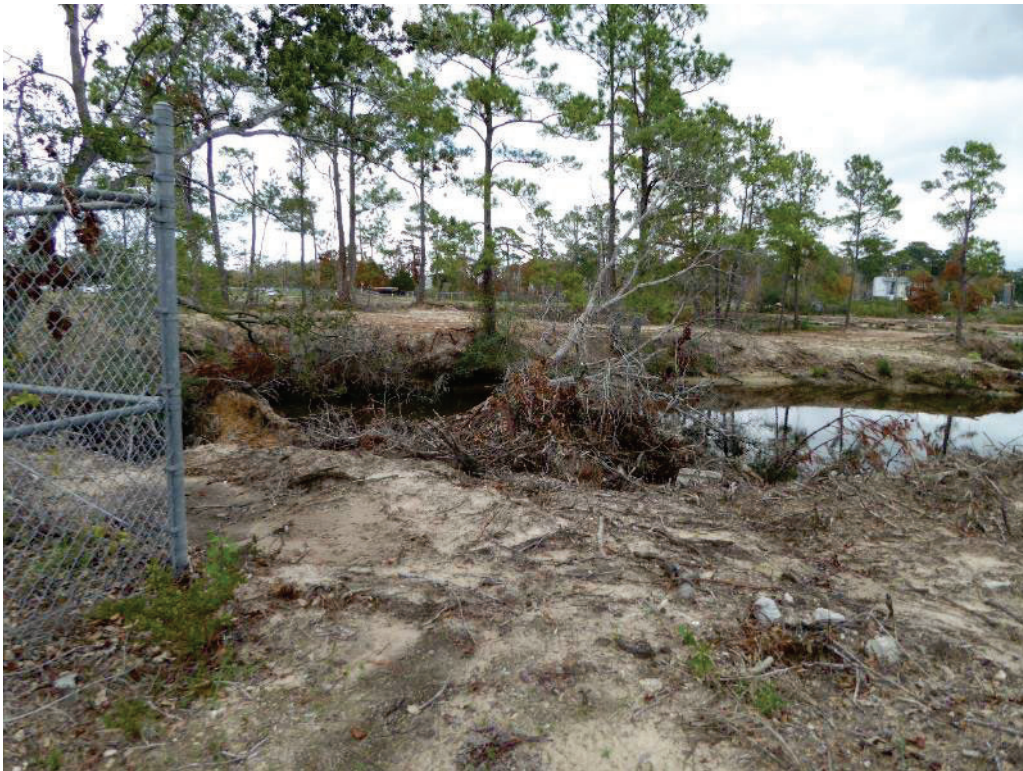
Cleared vegetation near the former sand pit
