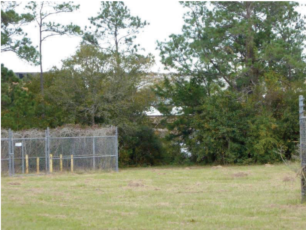
Monitoring well, with the Grennel Slough in background
