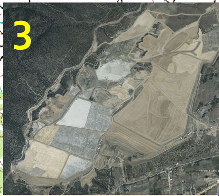
Tailing Facility Area
