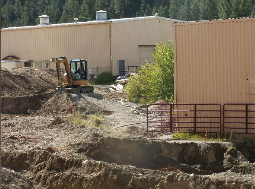
Soil Removal at Mill
