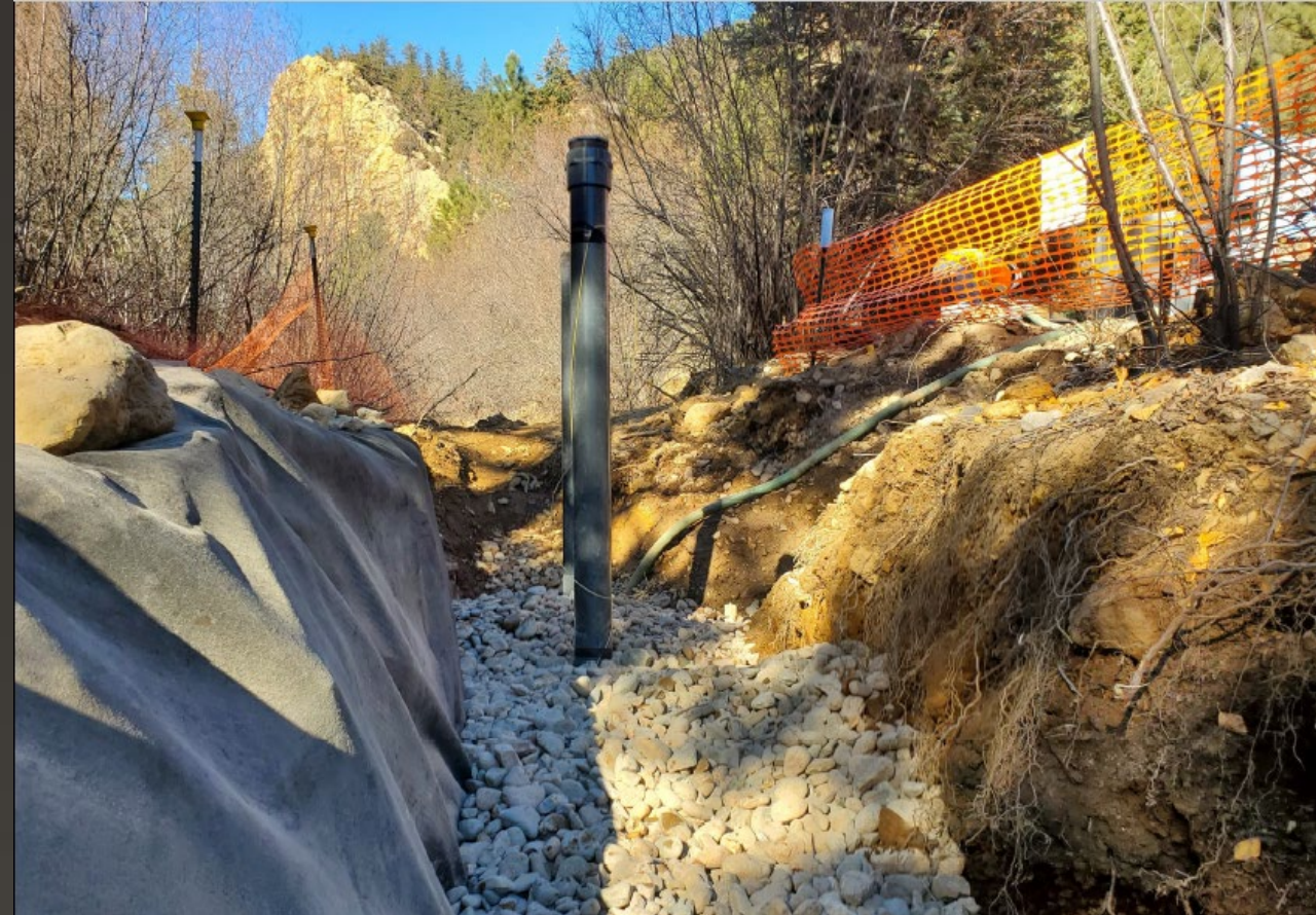
12/1: Installed cleanout, geotextile, and drain gravel within trench.
