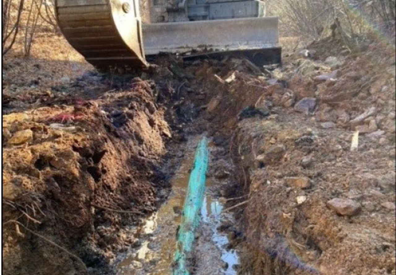
Excavated trench at STA 02+30.
