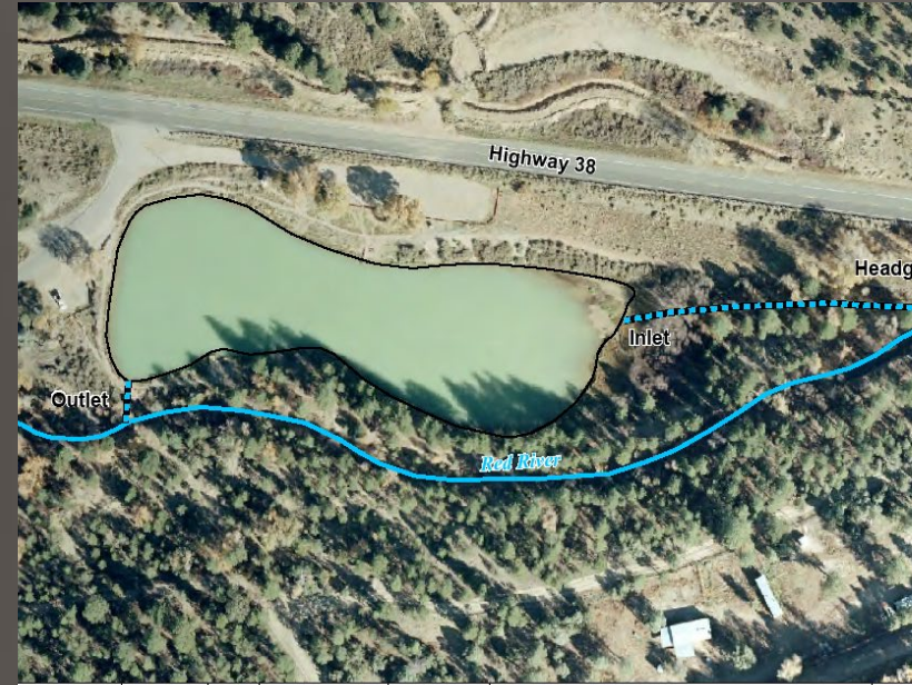
Eagle Rock Lake Before Removal
