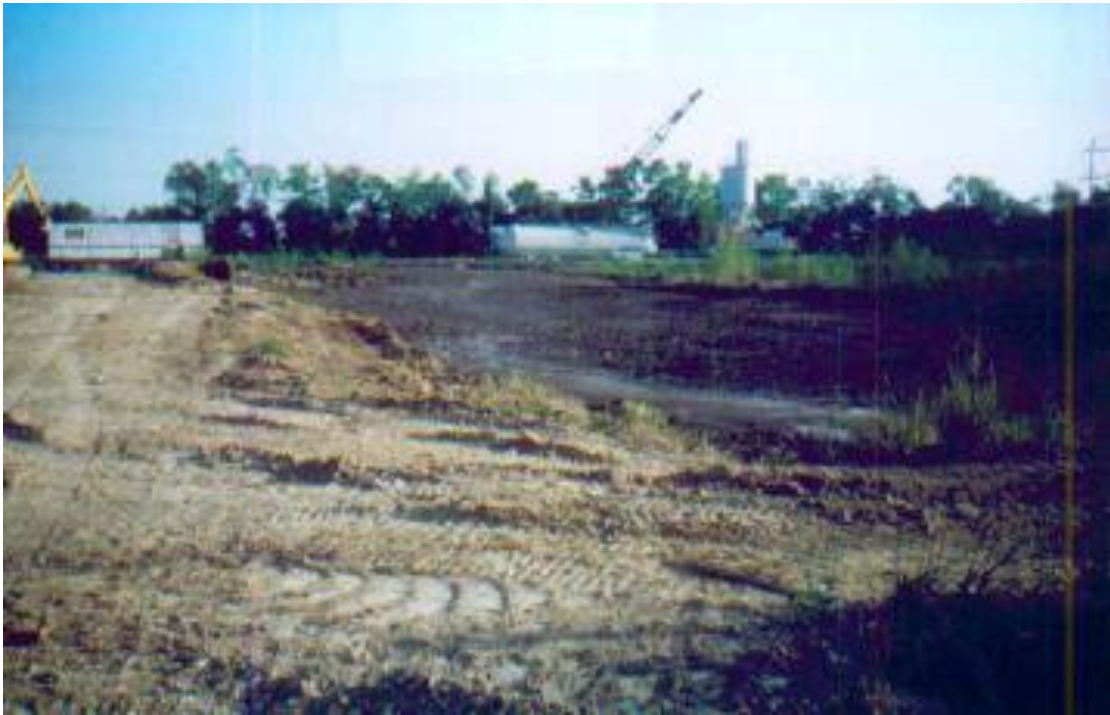
Dewatered pond area
