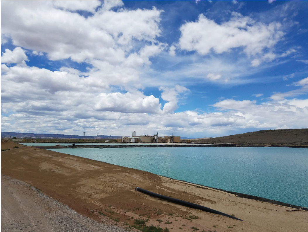
Collection ponds with RO treatment plant and LTP in the background, looking northwest
