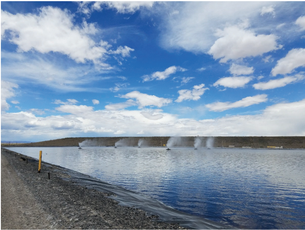
Evaporation pond 2 with sprayers
