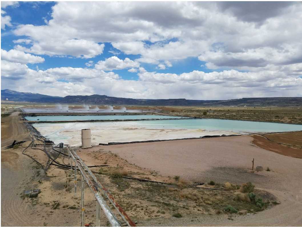
Collection ponds looking east from the RO treatment plant
