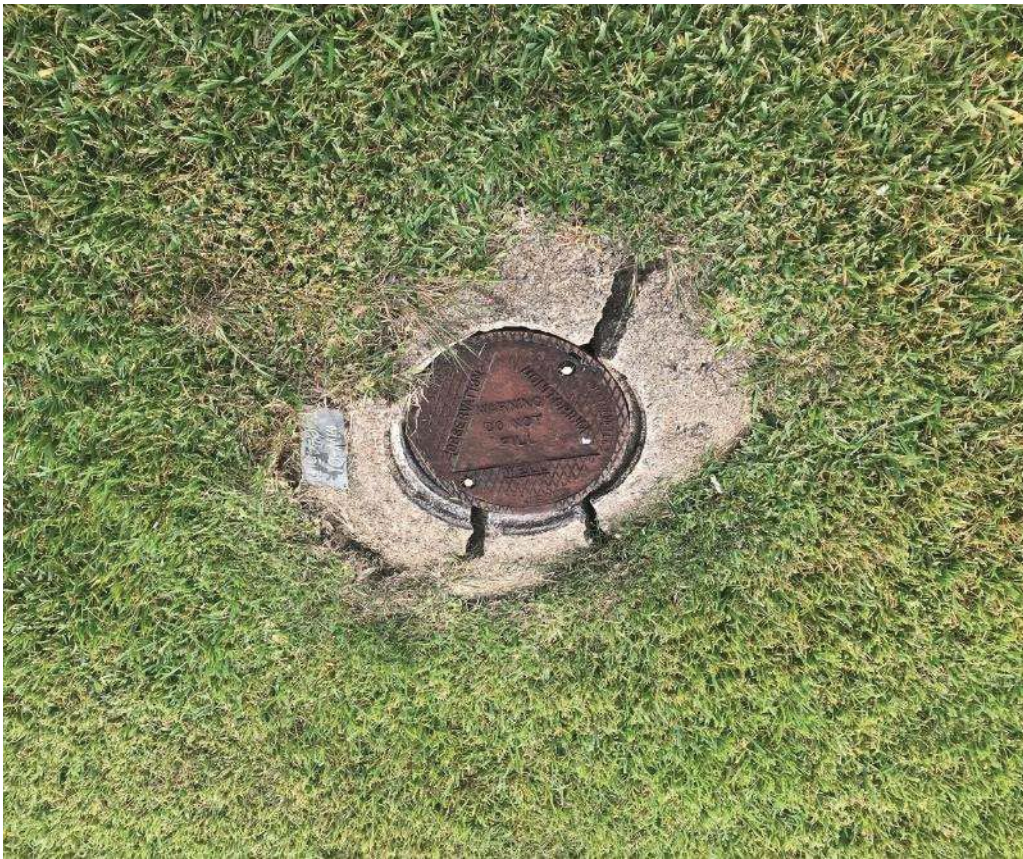
MW-01 with cracked well pad
