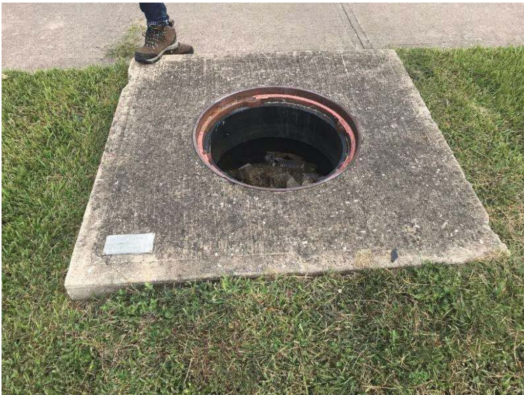
SZER-01 with missing manhole cover
