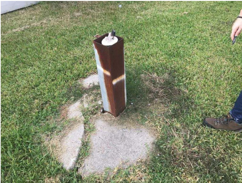
On-site well with missing steel lid and cracked well pad
