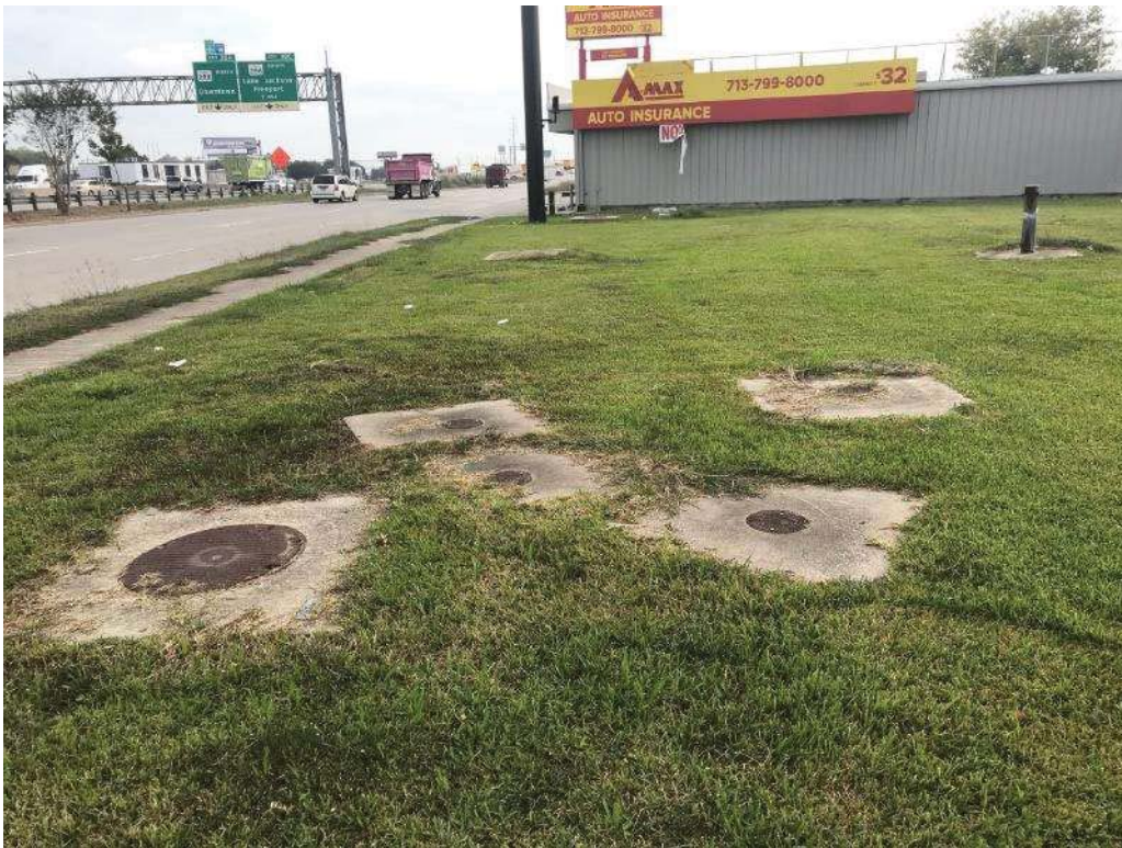
Monitoring wells and some recovery wells from previously operated groundwater treatment system, with businesses in background
