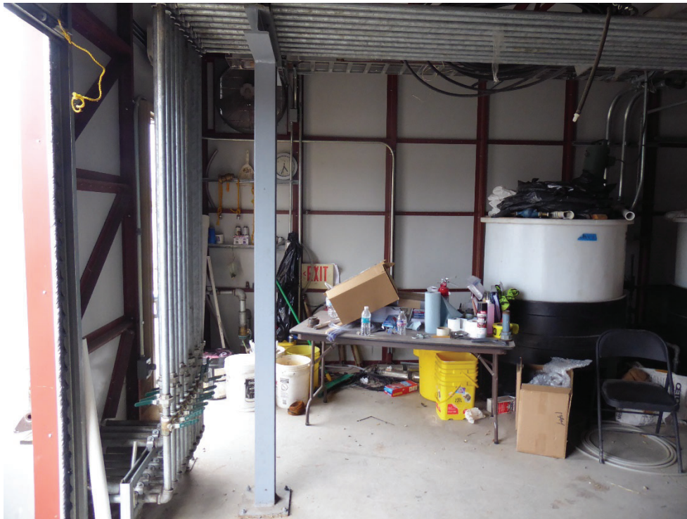
Photo 11: Interior of SA/HS building looking east from roll-up door entrance.
