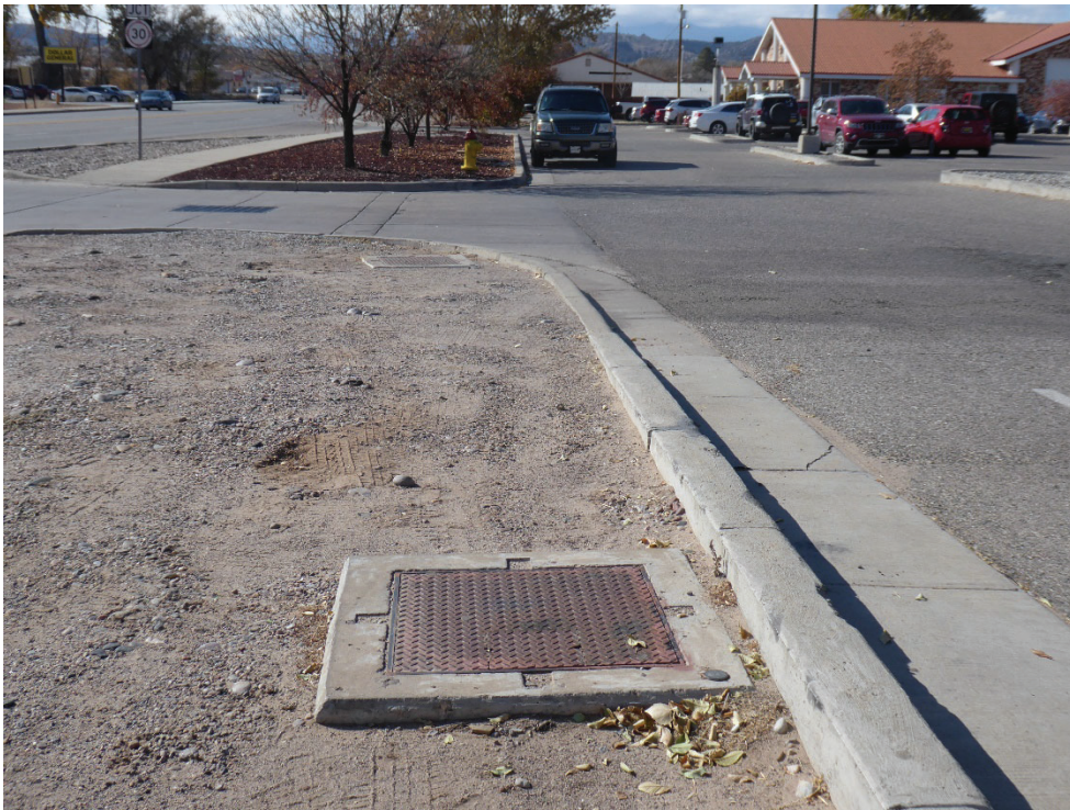
Photo 3: Biocurtain remediation well located south of La Cocina restaurant. Photo looking west.
