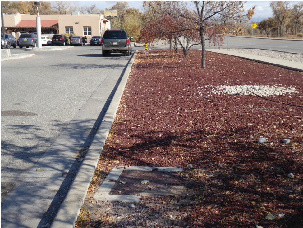
Photo 5: Biocurtain remediation well located east of La Cocina restaurant. Photo looking east.
