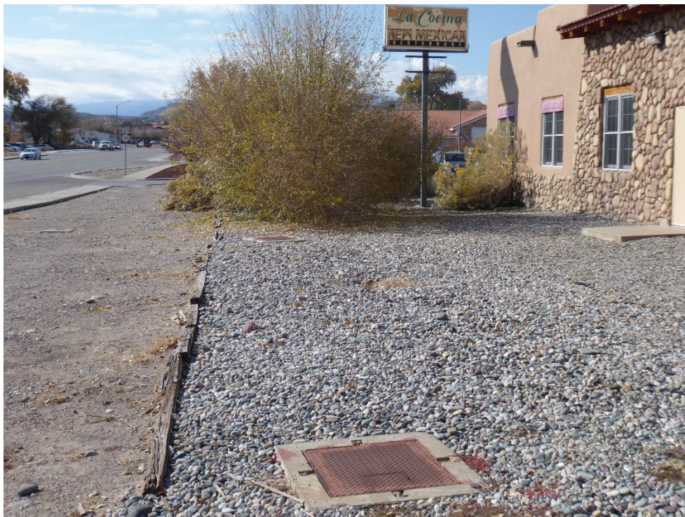
Photo 2: Biocurtain remediation well located southeast of La Cocina restaurant. Photo looking west.
