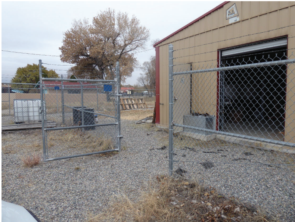
Photo 14: Normally locked access gate and SA/HS building. Photo looking east-southeast. Note location of hole in the fence (at white tote) that is shown in Photo 8.
