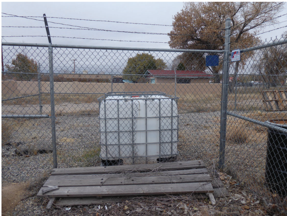
Photo 8: Existing (unrepaired) hole cut in the SA/HS Fence in the northeast end of the enclosure. Photo looking east.
