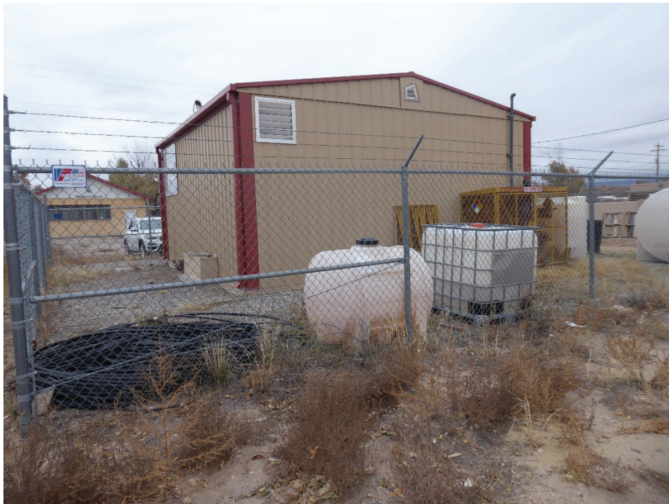
Photo 17: Southwest corner of the SA/HS Building, looking northeast.
