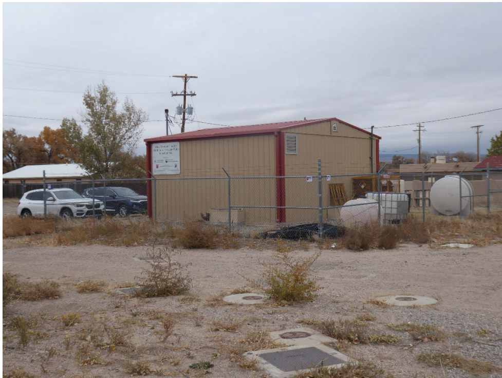
Photo 21: SA/HS building and enclosure with Source Area remediation and monitoring well vaults in the foreground. Photo looking northeast.
