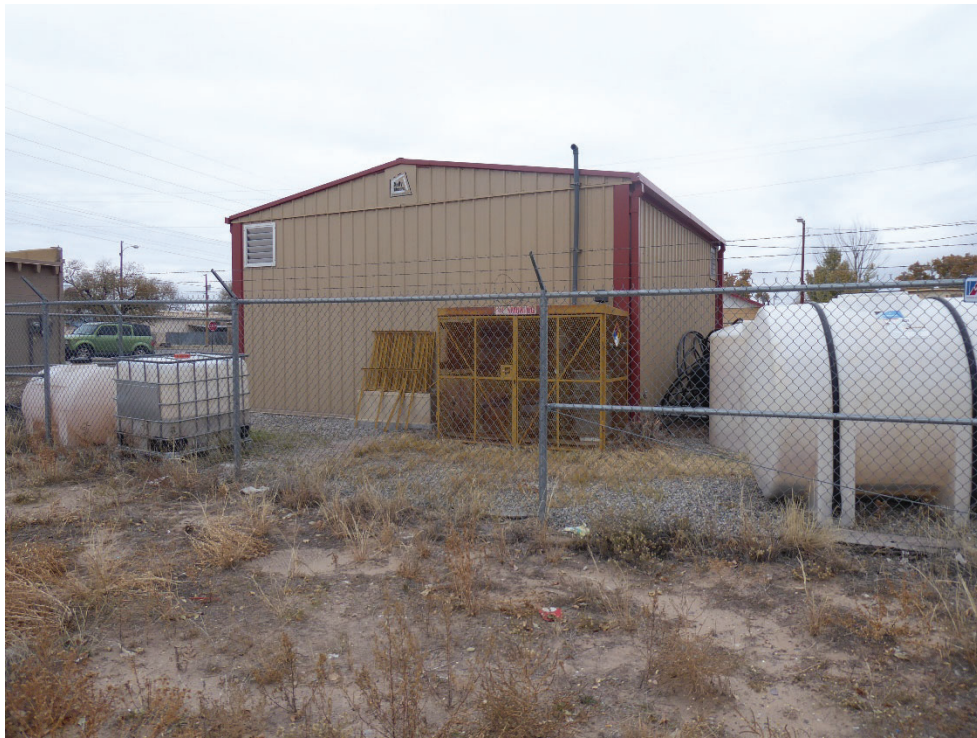
Photo 15: South side of the SA/HS building and enclosure. Photo looking northwest.
