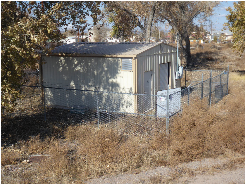
Photo 1: Biocurtain Building. Photo looking north.
