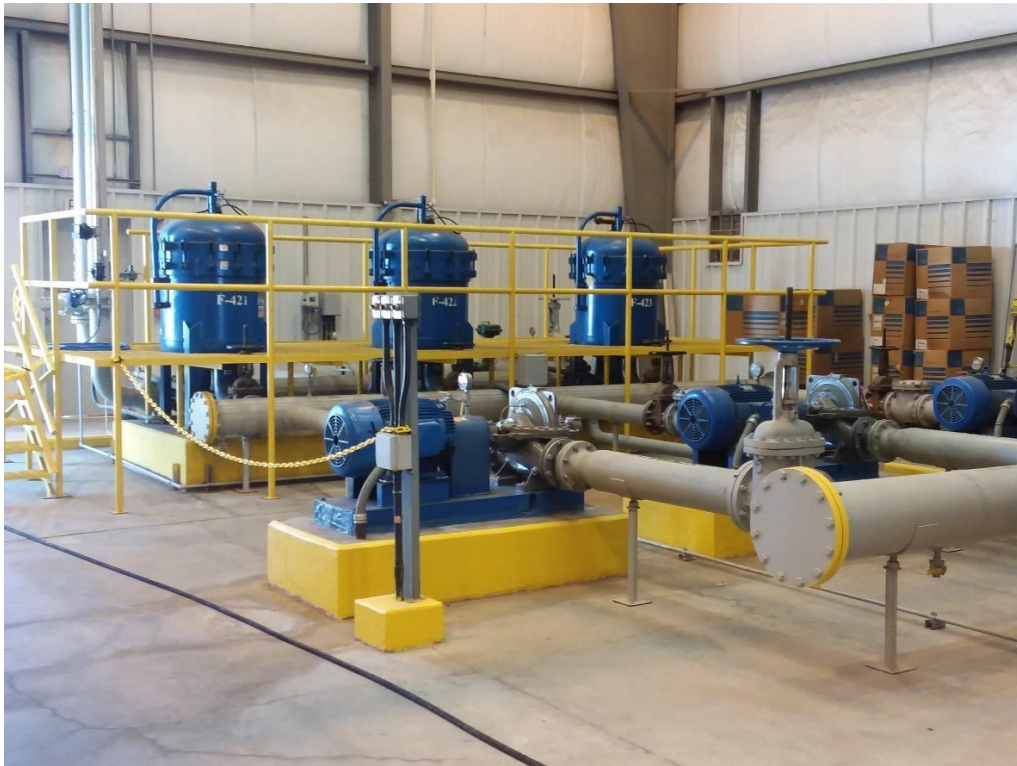
Photograph No. 19 Site: South Valley Superfund Description: OU 06, Injection Pumps and Filters. Treated Water is pumped to Injection Wells.
