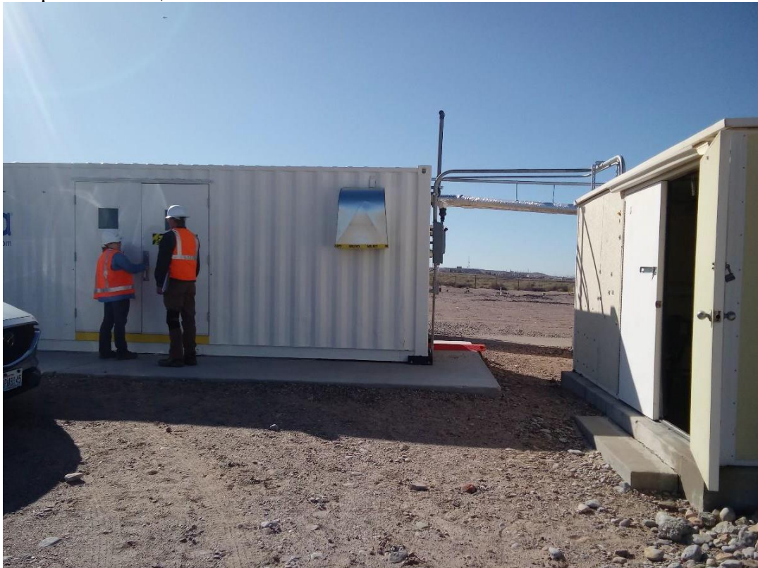
Photograph No. 3 Site: South Valley Superfund Description: OU 03, New 1,4-dioxane Advanced Oxidation Treatment Building.
