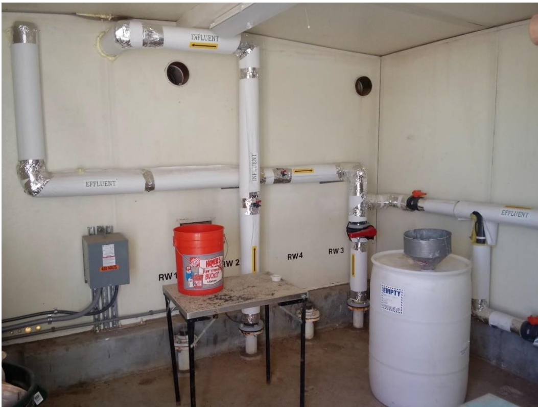
Photograph No. 2 Site: South Valley Superfund Description: OU 03, Extraction Wells Influent and effluent from Old Treatment Building.
