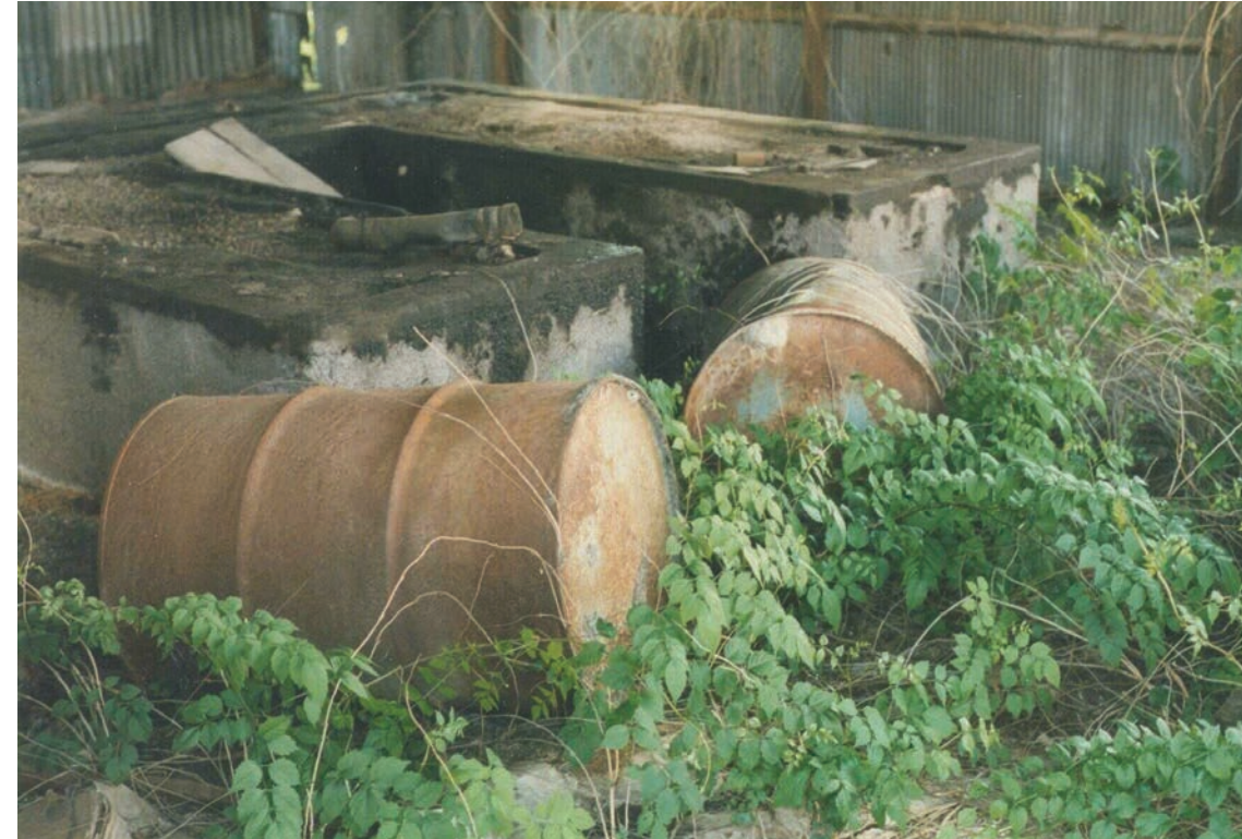
Building #15 at the Eagle-Picher complex.
