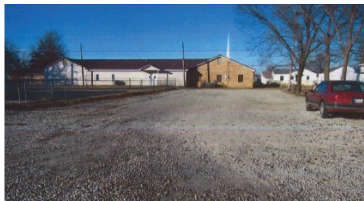
Ongoing OU2 actions include sampling high-access areas such as this church parking lot.
