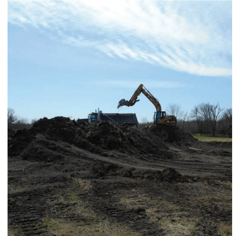
Cleanup of Chat Pile CP009.
