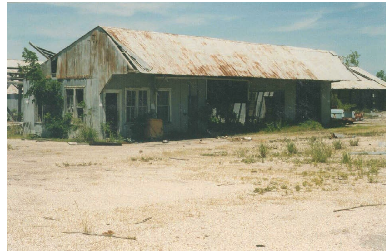
Building #13 at the Eagle-Picher complex.
