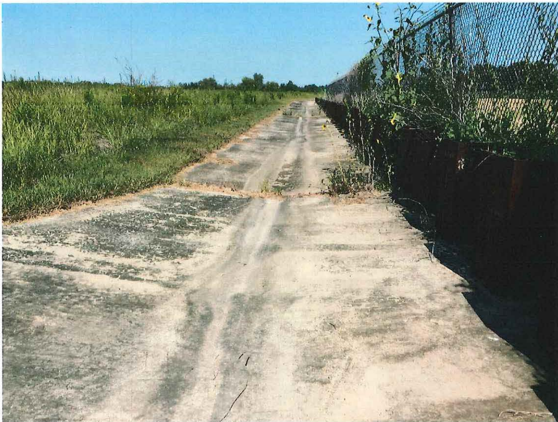
Brio North Sheet Pile Barrier Wall and Drainage Road Looking Southeast
