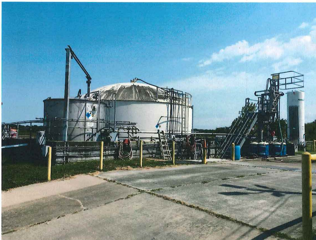
Recovered Groundwater and DNAPL Storage Tanks
