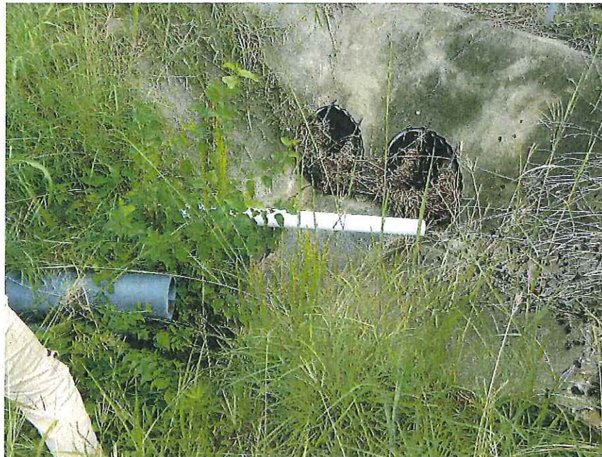
Effluent discharge outfall piping
