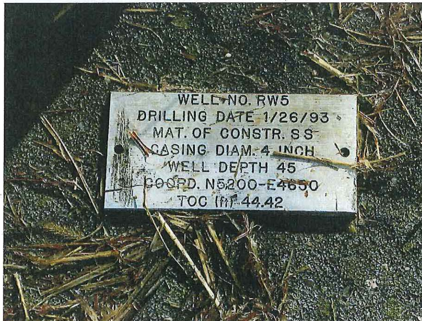
Clearly marked recovery well RW-5
