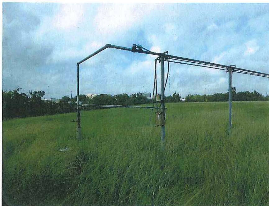
Piping, part of the active groundwater recovery and treatment system
