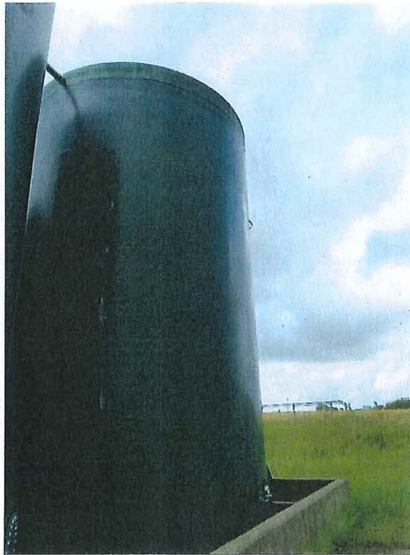
One of the six tanks where treated groundwater is stored before discharge
