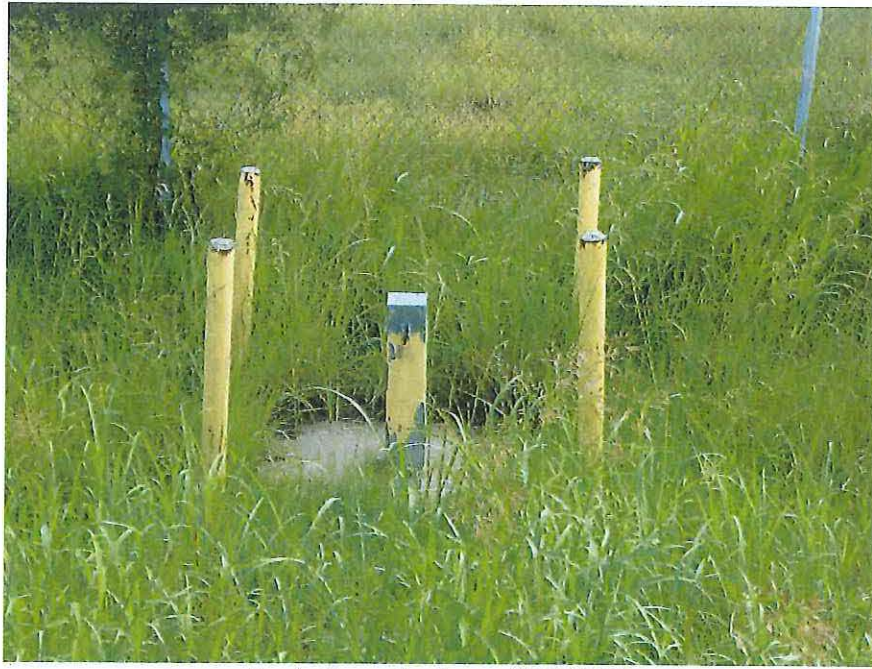
Locked monitoring well MW-26
