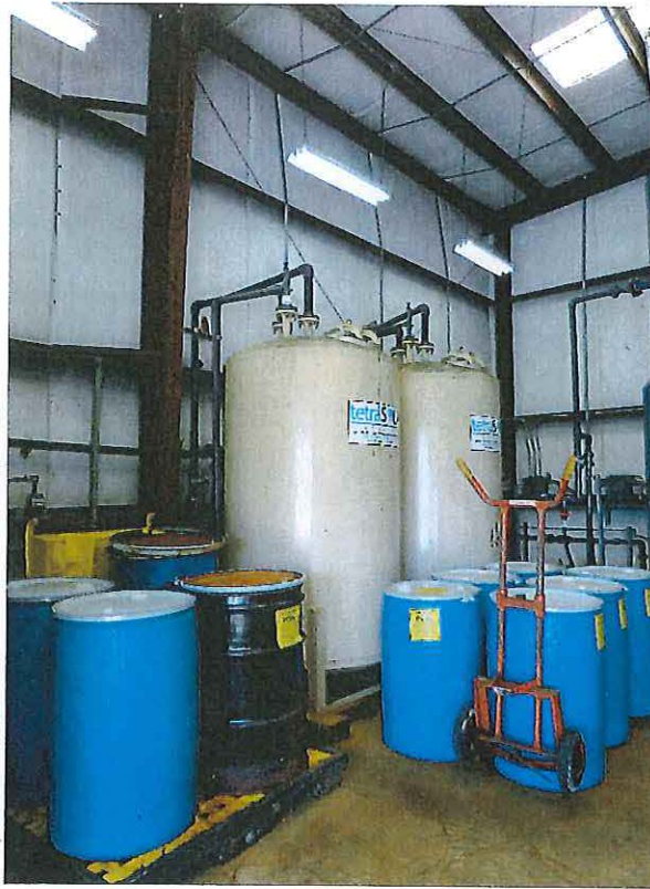
Granular activated carbon tanks, part of the groundwater recovery and treatment system
