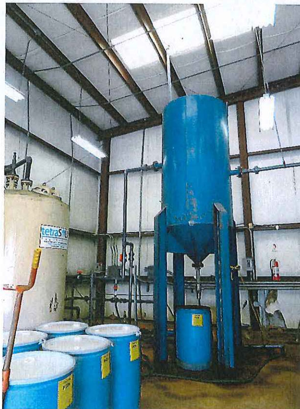
Oil/water separator tank, part of the groundwater recovery and treatment system
