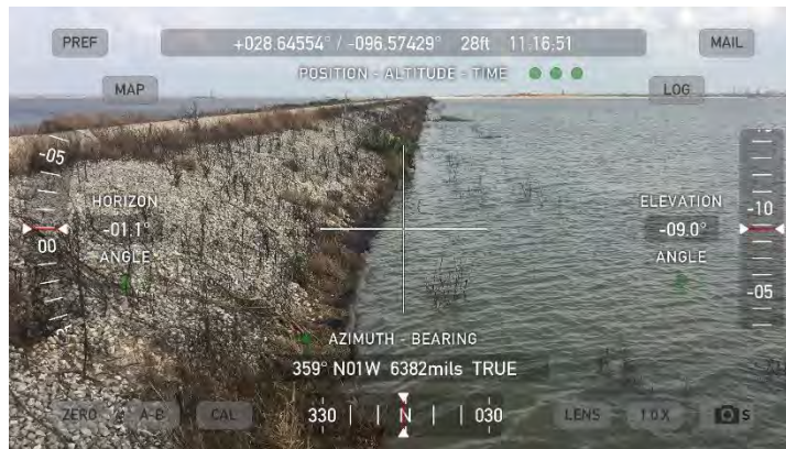
West Dike, Interior, Minor Erosion at Toe (facing north)
