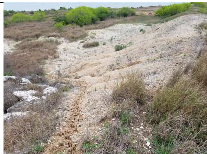
33 – East CPA Outer Dike, viewing erosion
