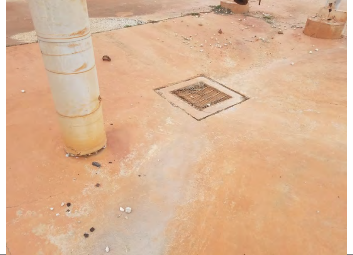
2 - Cap, storm sewer drain at R-301
