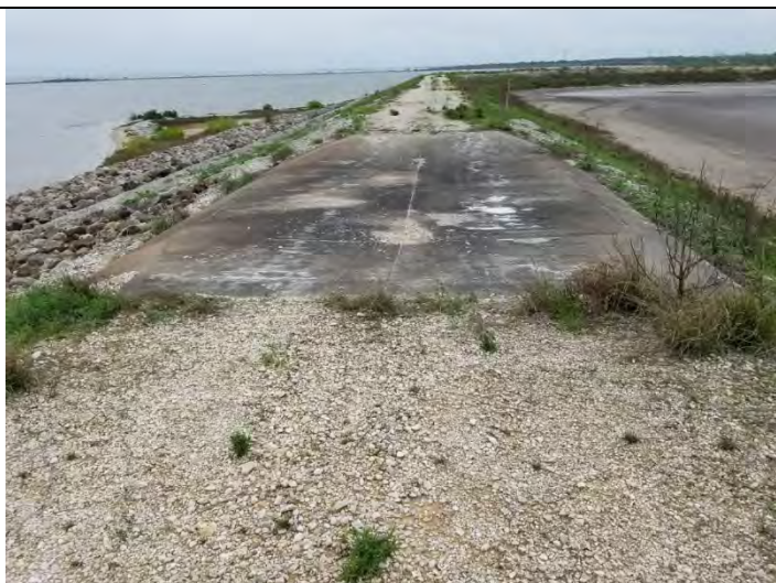
30 – Emergency Spillway, viewing minor deterioration of the concrete and surrounding vegetation
