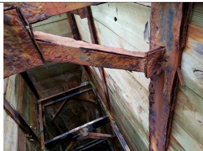
35 – View North Decant Structure deterioration
