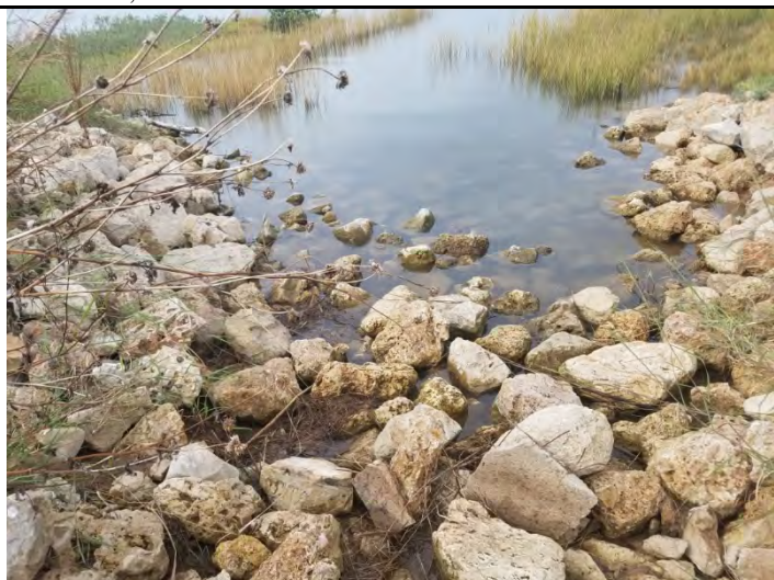
14 – Drainage channel, West end of new channel, view rip rap to bay
