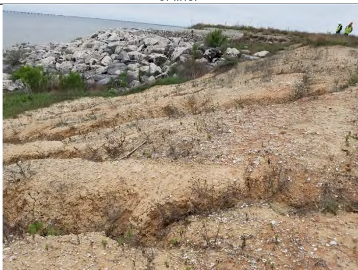
34 – West CPA Outer Dike, viewing erosion
