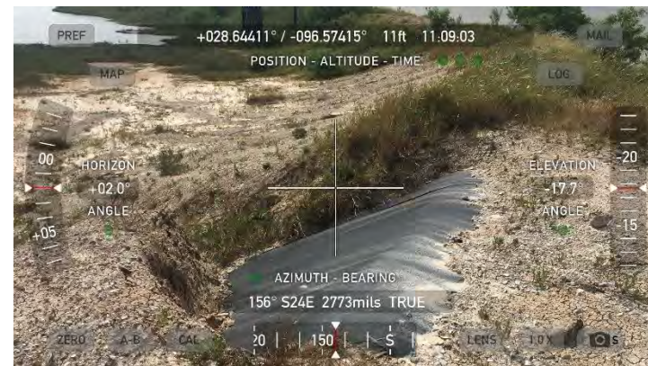
Port CDF Erosion/Exposed FML at West Water Stop – Interior Slope
