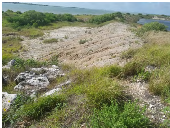
33 – East CPA Outer Dike, viewing erosion
