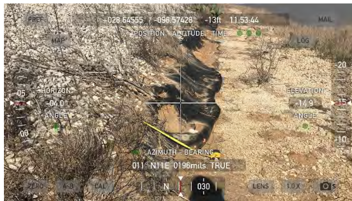
West Dike Interior Erosion (facing north)
