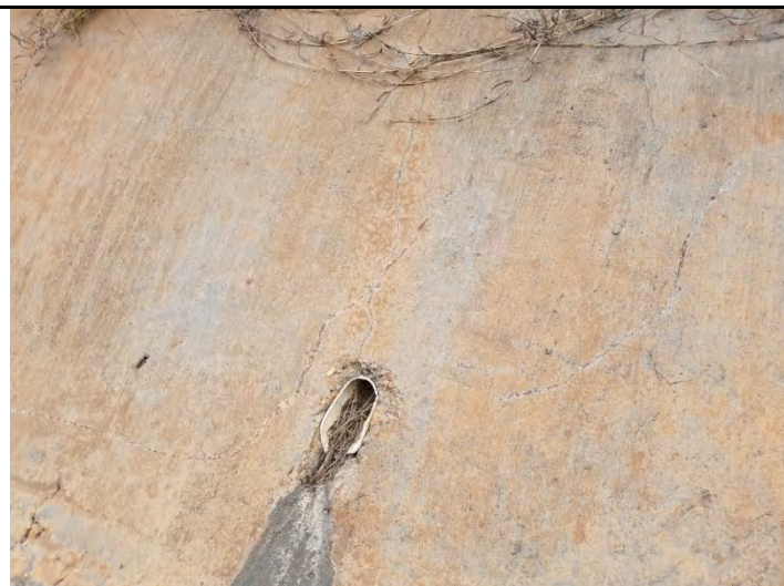
13 – Drainage channel, viewing drainage pipe into channel
