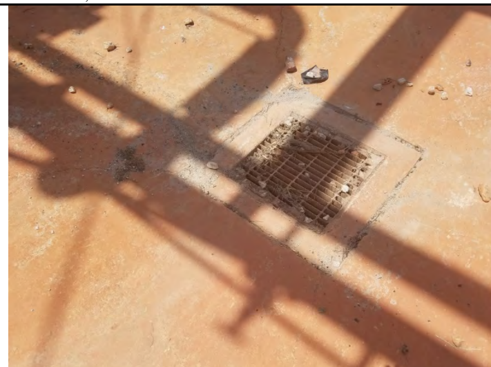
2 - Cap, storm sewer drain at R-301
