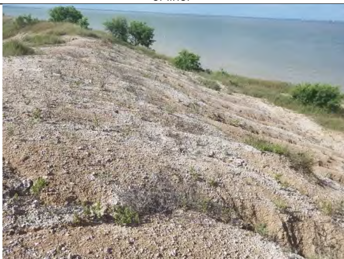
34 – West CPA Outer Dike, viewing erosion
