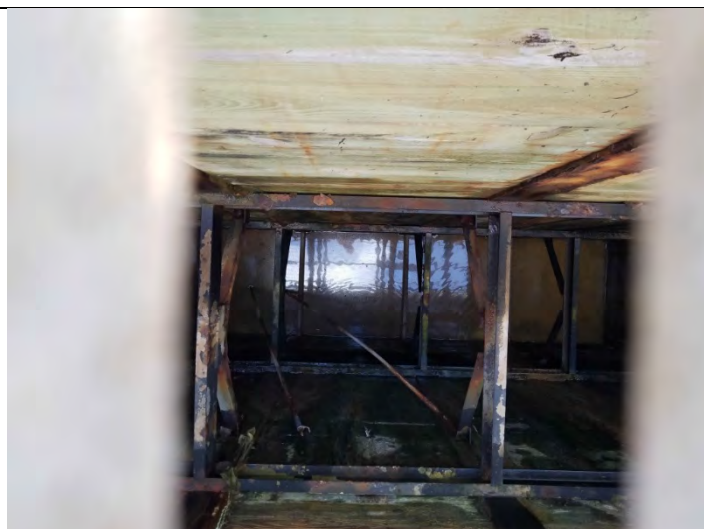
35 – View North Decant Structure deterioration
