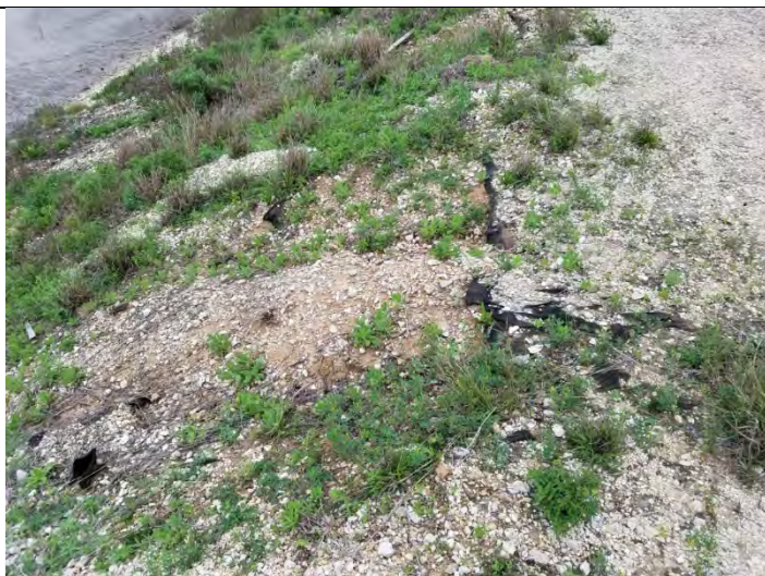
4 – North Inner Dike, viewing minor erosion and geofabric exposure
