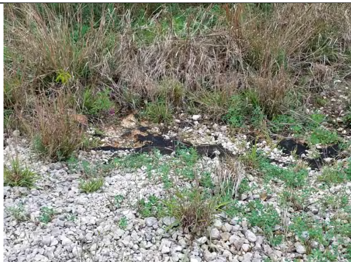
19 – South Dike, viewing exposed geomembrane
