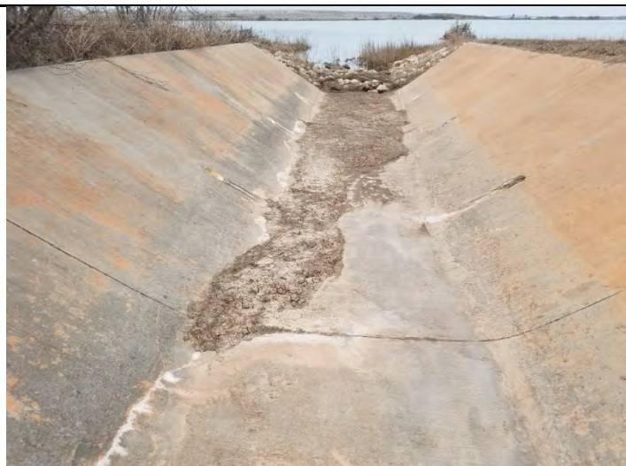
23 – Drainage Channel, viewing sediment buildup at West end of channel
