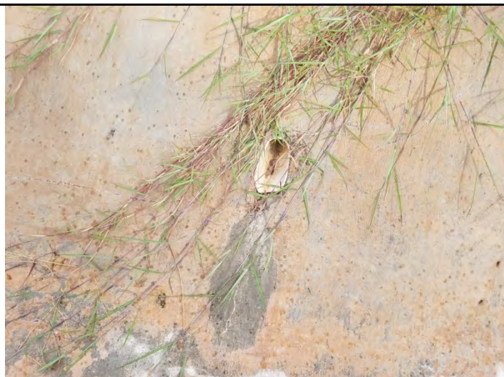
13 – Drainage channel, viewing drainage pipe into channel
