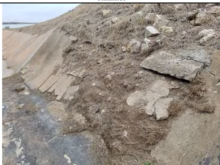
10 – Drainage channel, viewing deterioration of old channel
