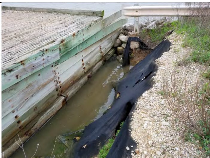
36 – Dredge Island Access Bridge, viewing erosion between the bridge and the island
