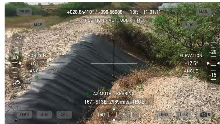
Port CDF Erosion/Exposed FML at East Water Stop – Interior Slope
