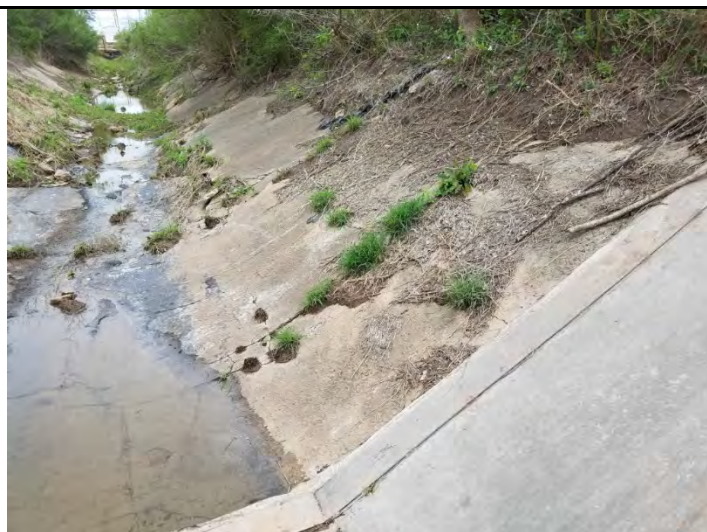
10 – Drainage channel, viewing deterioration of old channel
