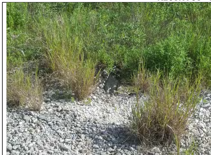
19 – South Dike, viewing exposed geomembrane
