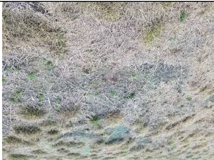
20 – Slope from cap to channel, viewing bare spot and exposed geofabric
