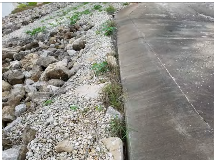
29 – Emergency Spillway, viewing minor erosion along outer edge
