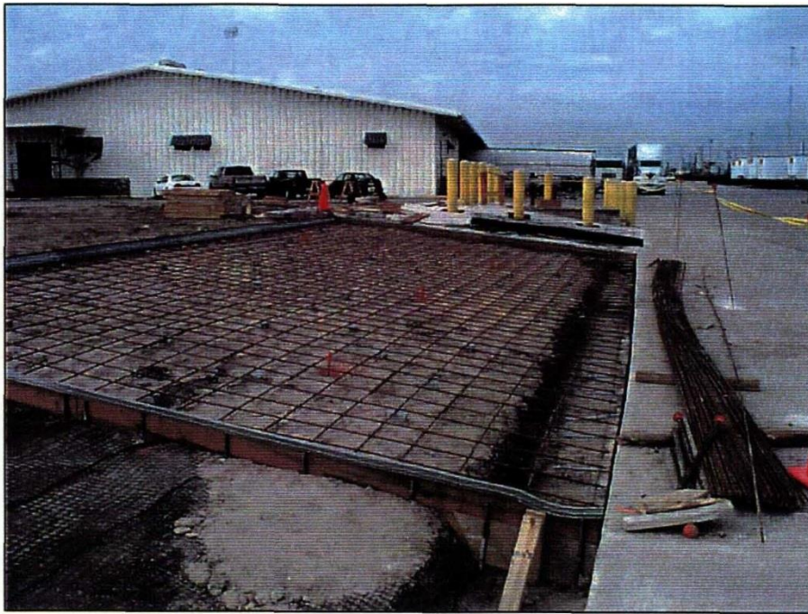
PHOTOGRAPH 3: REBAR PLACEMENT AND THICKENED EDGE IN SOUTHWEST AREA
