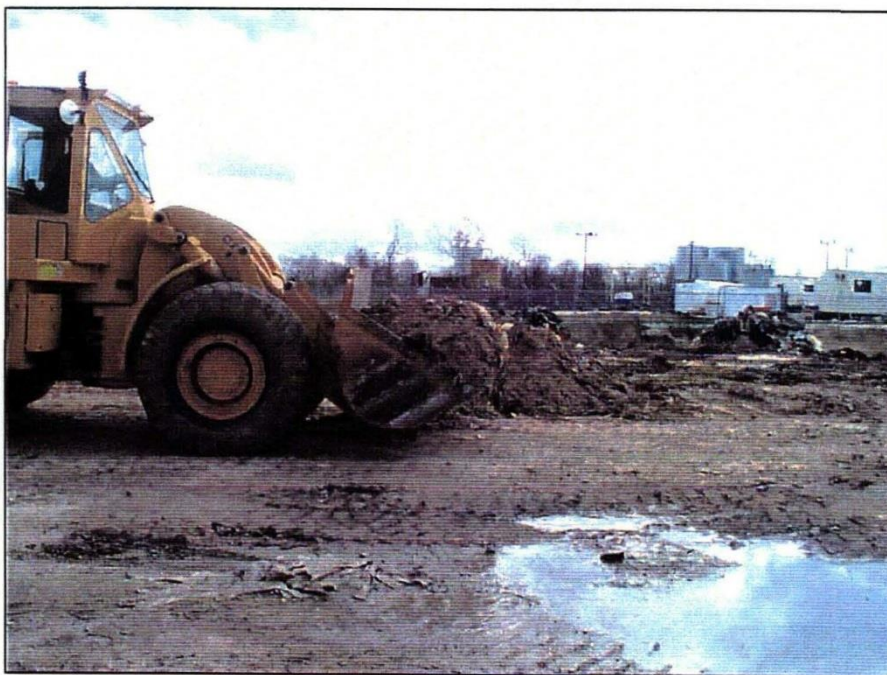
PHOTOGRAPH 2: STOCKPILE 12 HAULING FOR FILL
