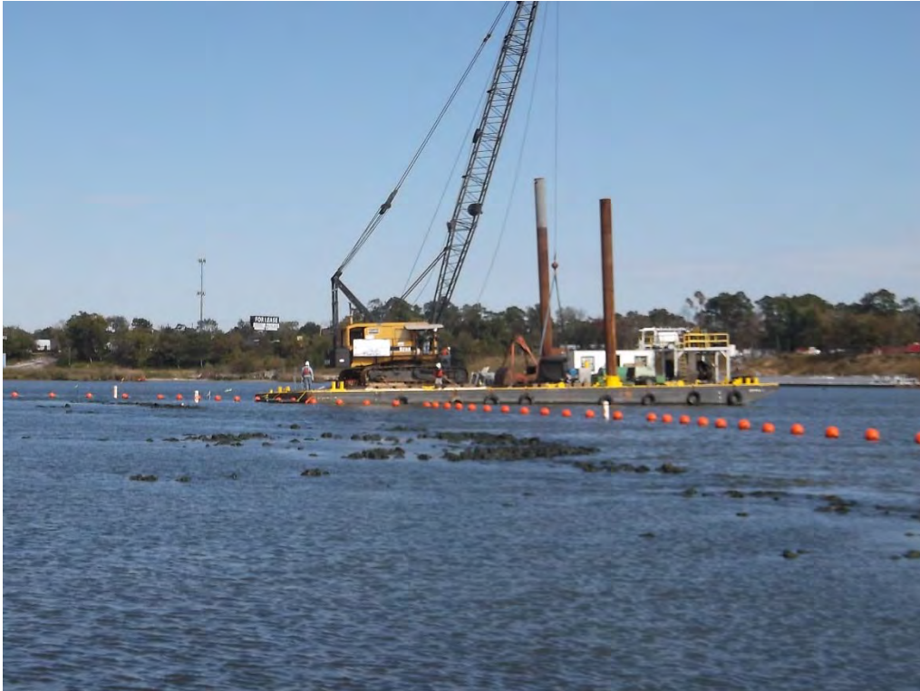
Photograph 2: Orion deck barge spudded down at the slope improvement area
