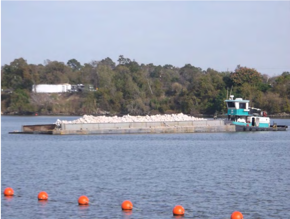
Photograph 4: Arrival of D rock aggregate to the site.
