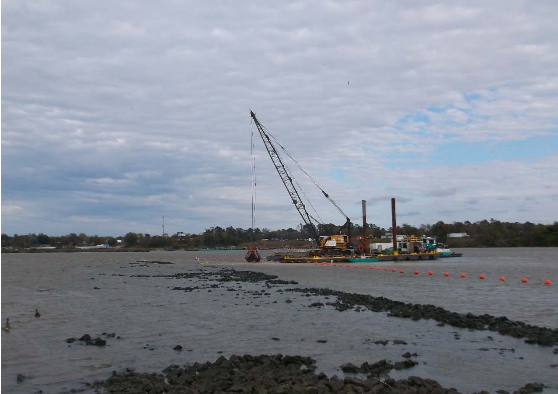
Photograph 2: Orion work barge placing stone near south end of maintenance area
