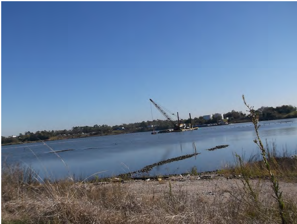
Photograph 3: Orion placing rock on panels 1 and 2 for the day (panels 7 and 8 for the job)
