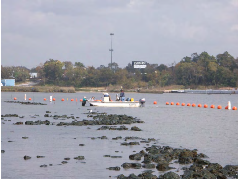
Photograph 1: HCL installing stakes along proposed geotextile edge
