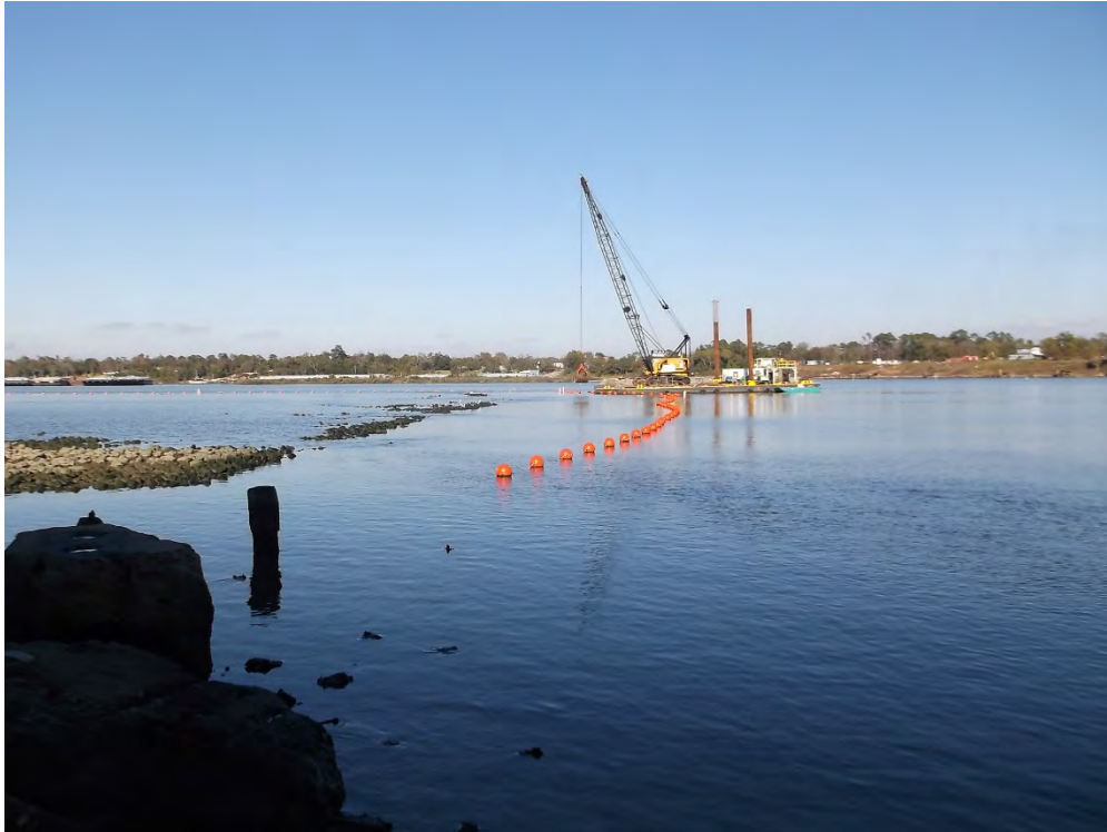
Photograph 4: Orion placing rock on panels 1, 2 and 3 for the day (panels 7 to 9 for the job)
