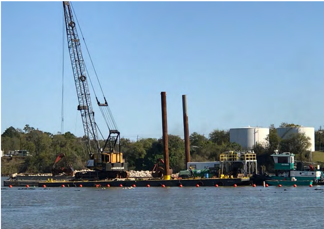
Photograph 2: Orion placing rock
