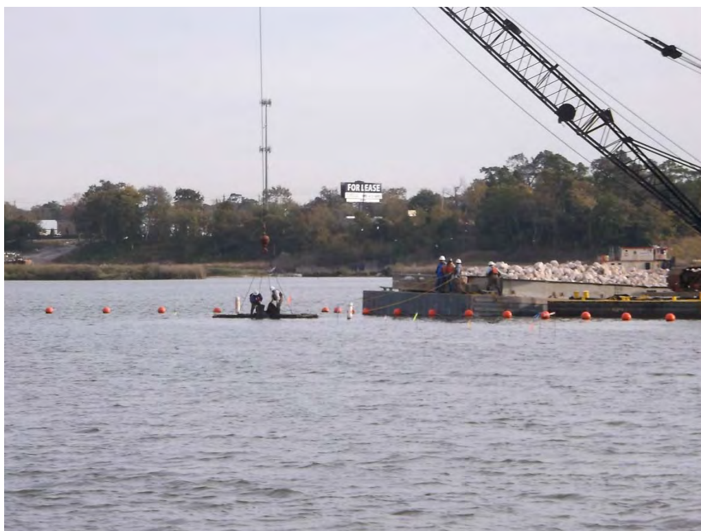
Photograph 1: Orion deck barge, rock barge and geotextile crew.
