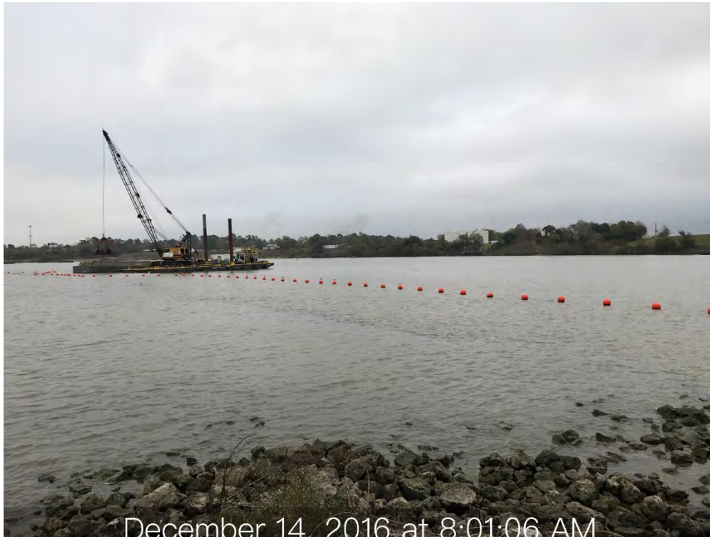
Photograph 1: Orion work barge placing stone near south end of maintenance area
