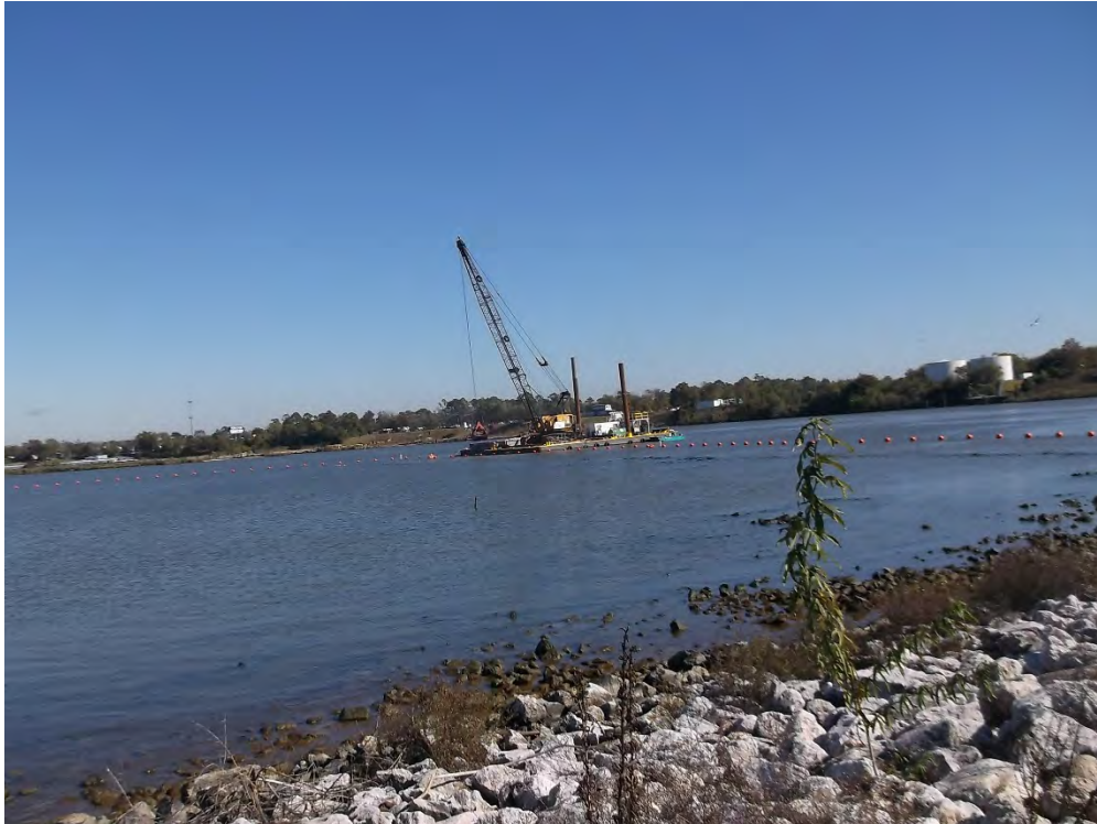
Photograph 2: Orion work barge placing stone
