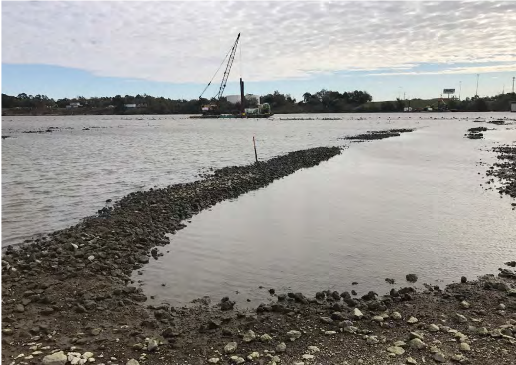
Photograph 1: Orion work barge placing stone near south end of maintenance area
