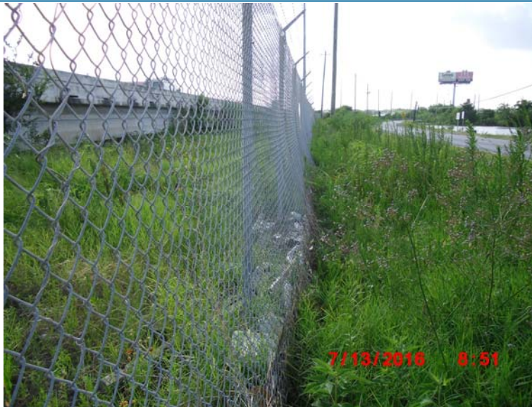
Photograph 17: Perimeter fence located south of I-10 on west bank that was damaged during recent floods (view east)
