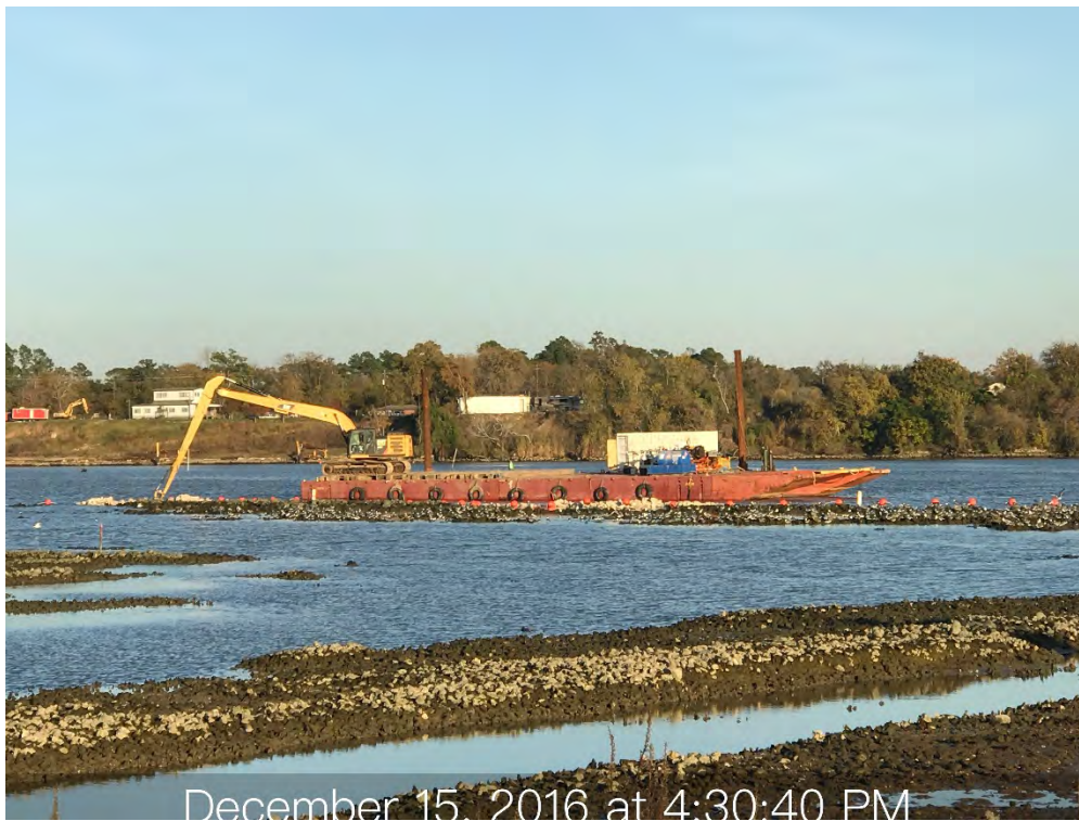
Photograph 3: Excavator shaping rock areas.
