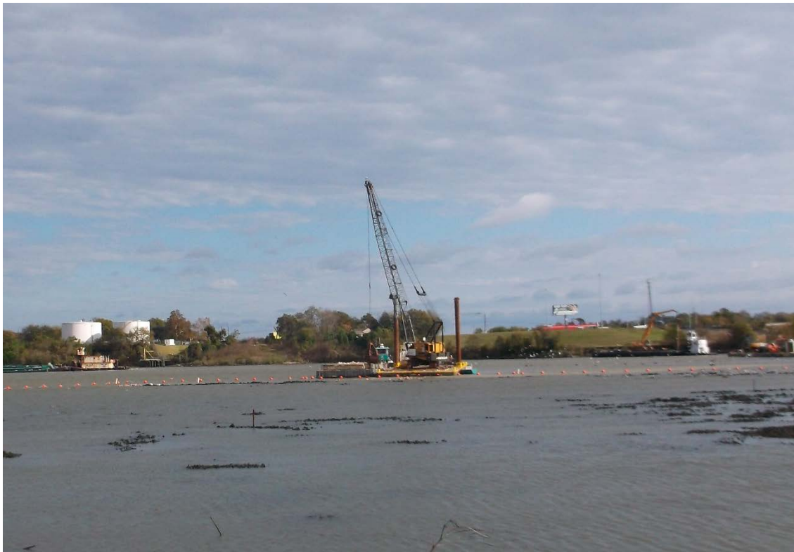
Photograph 3: Orion placing rock thickness during low tide
