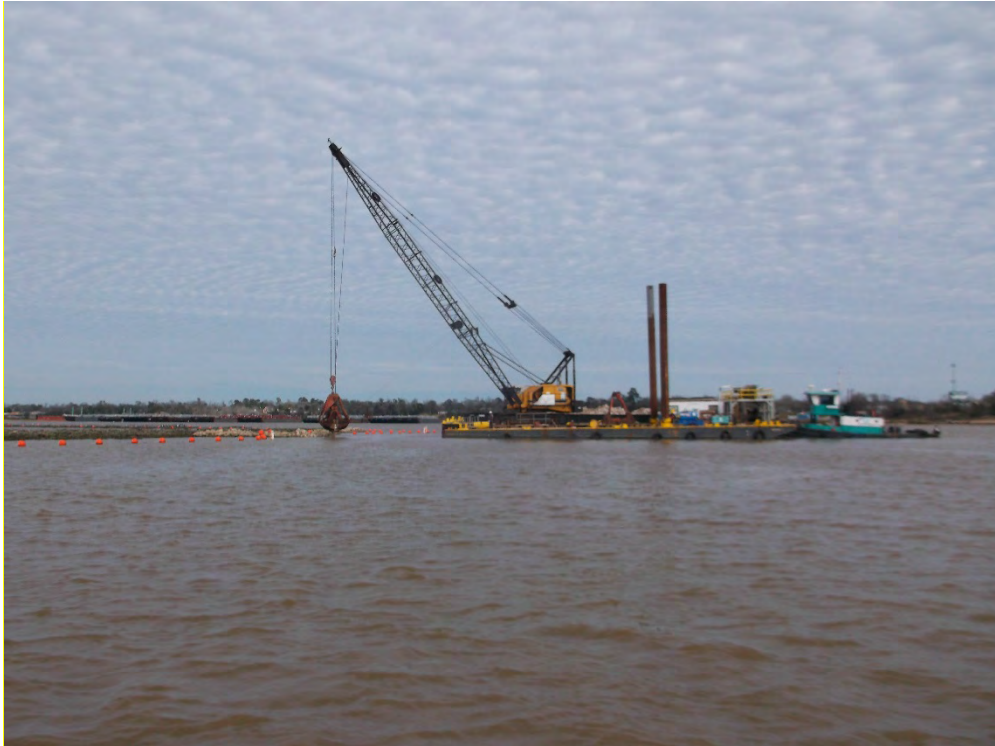
Photograph 2: Orion work barge placing stone near south end of placement area
