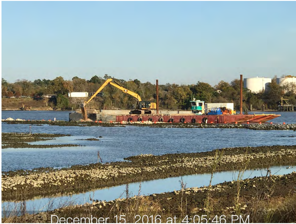
Photograph 2: Orion work barge placing stone near south end of maintenance area
