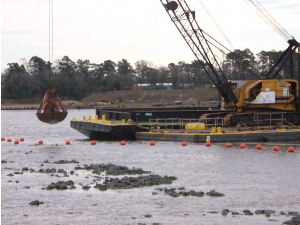
Photograph 1: Orion work barge placing stone near south end of placement area.
