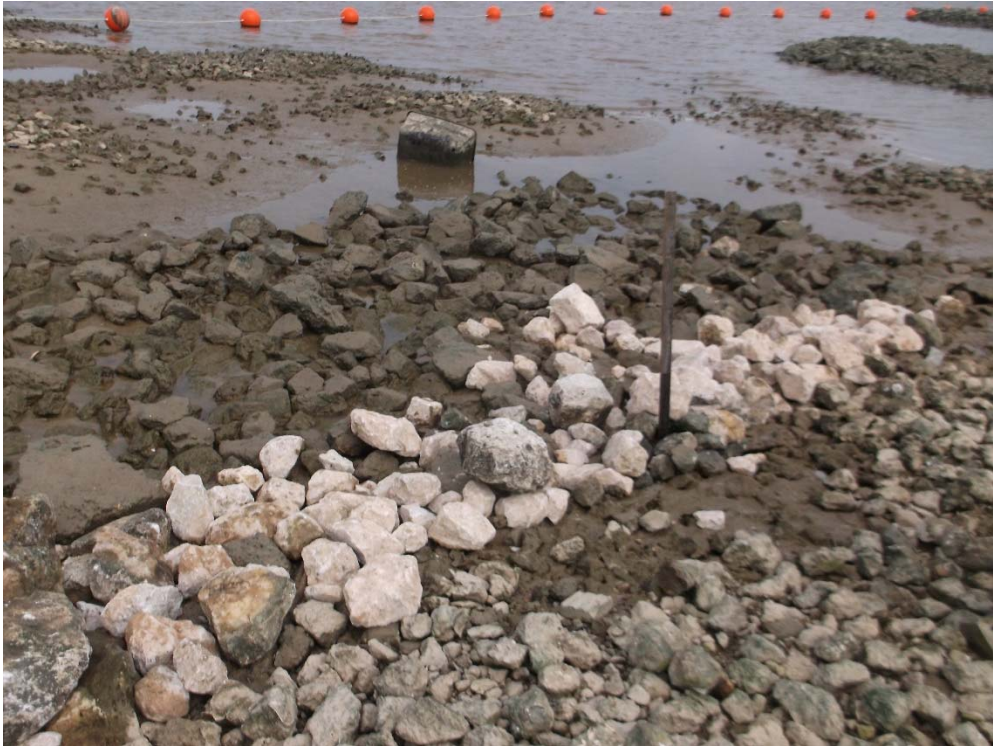
Photograph 4: View of a western cell location after rock placement.
