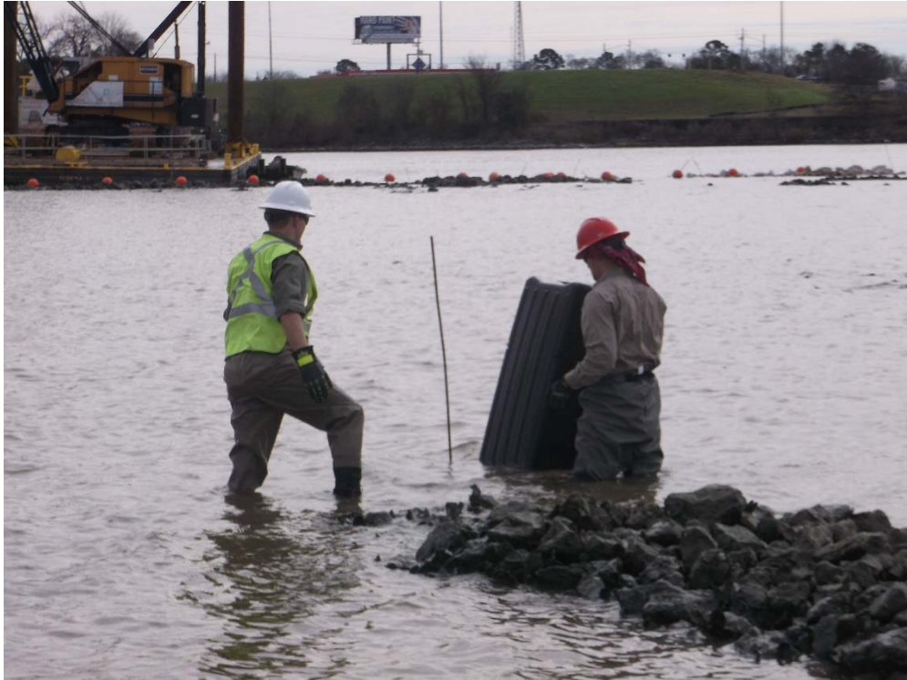
Photograph 2: Placing C rock on maintenance location 3.
