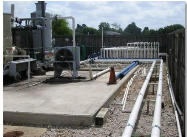
Figure 4. On-site LNAPL extraction and treatment system.
