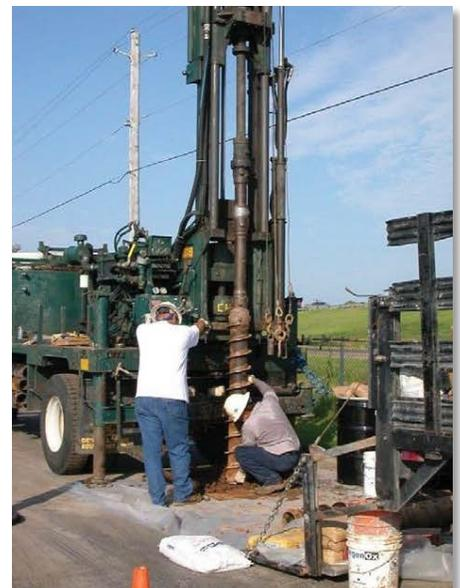
**Figure 2. Well installation during remedy construction.**
