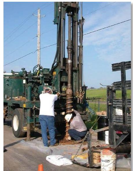
**Figure 2. Well installation during remedy construction.**
