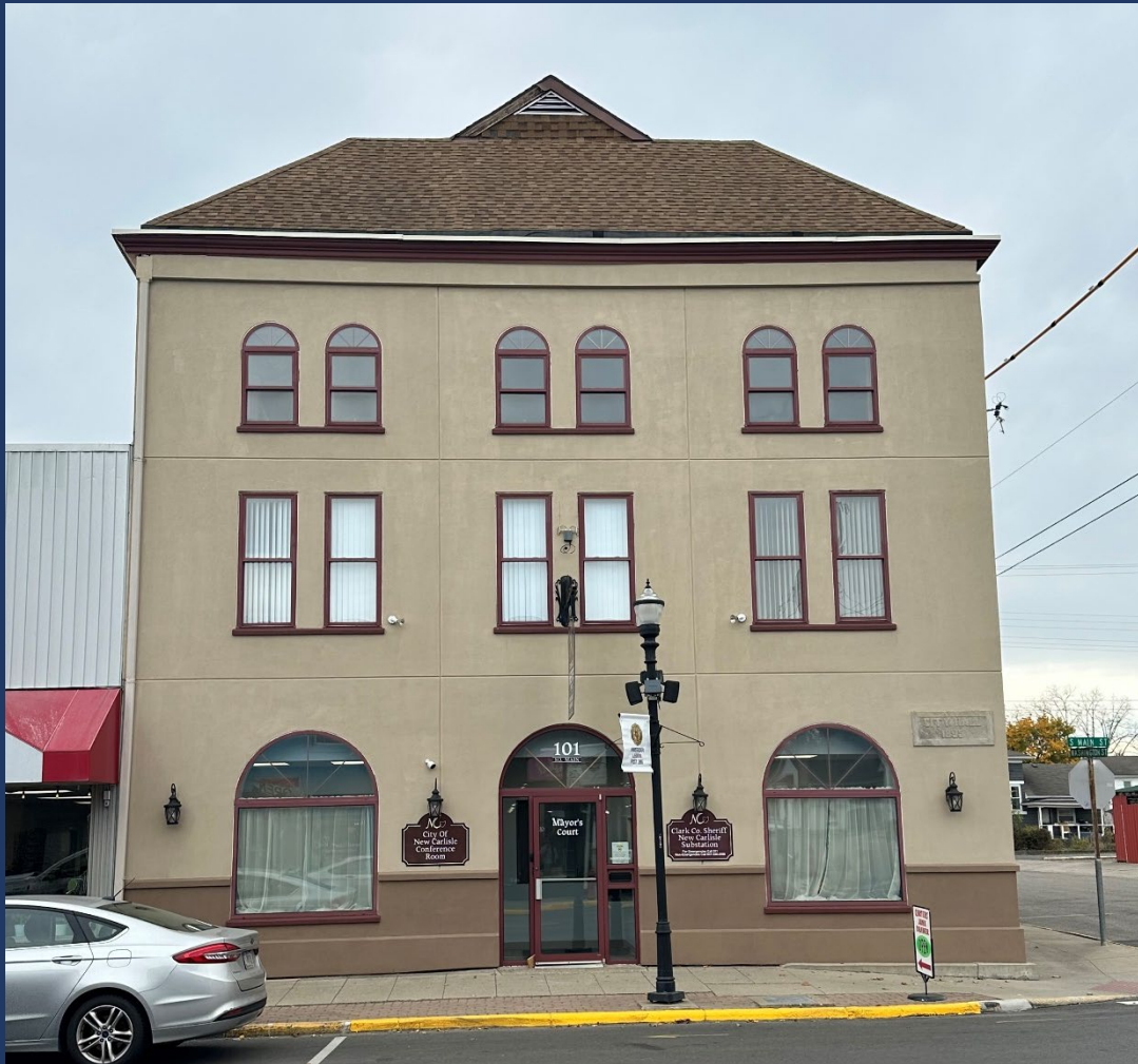
City of New Carlisle Conference Room, Mayor's Court and Clark County Sheriff New Carlisle Substation at 101 South Main Street.
