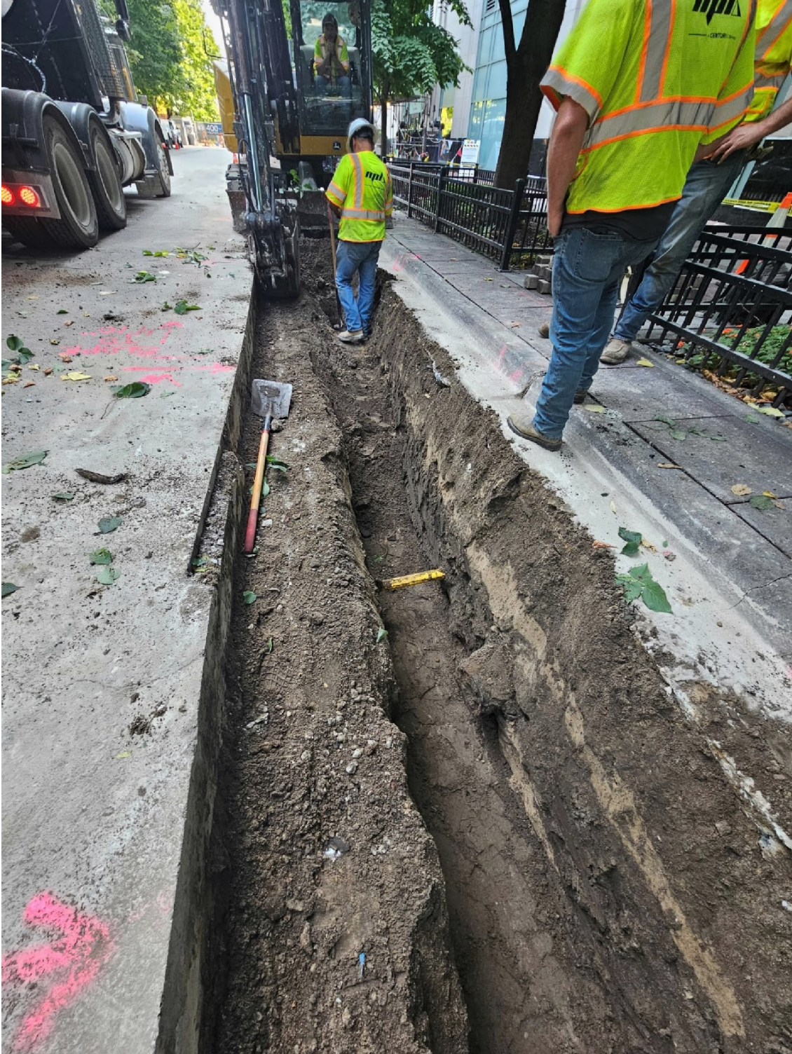
PICTURE 4: VIEW OF EXCAVATION RUNNING EAST ALONG E NORTH WATER STREET.
