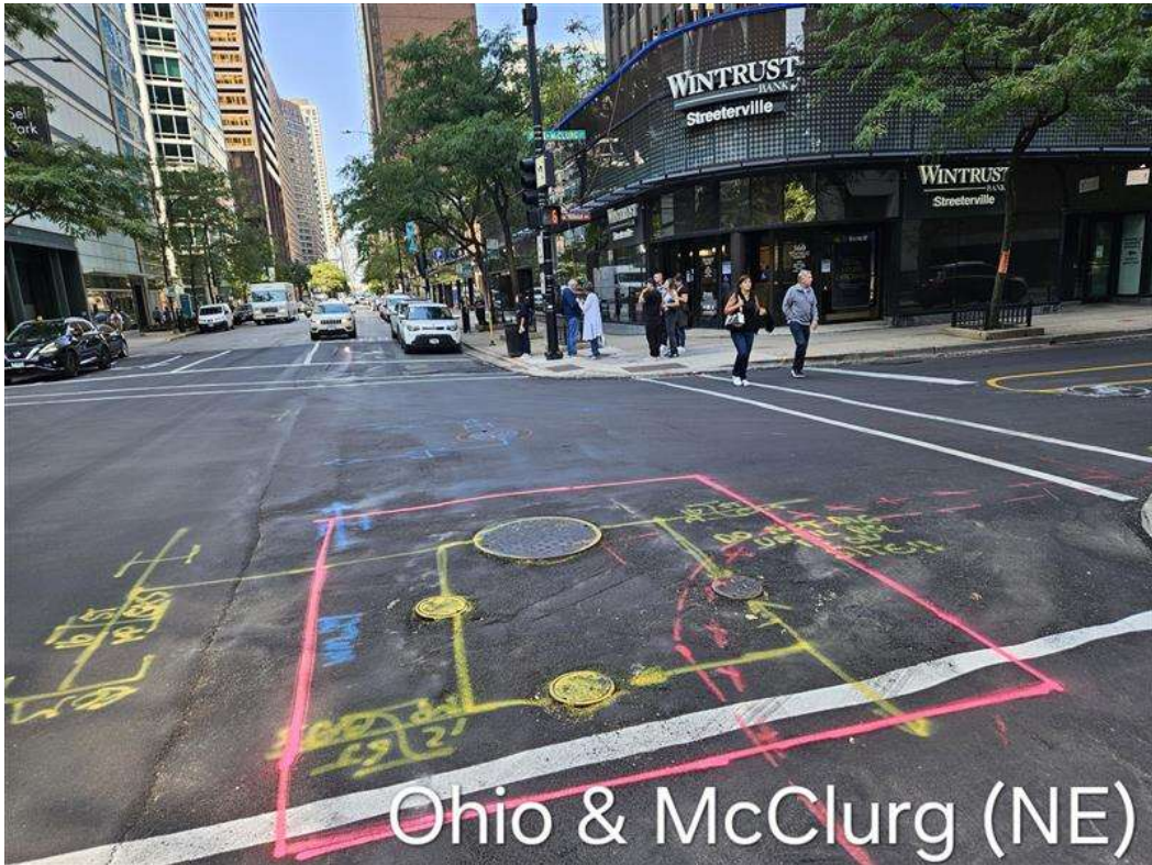
PICTURE 13: DOT1992955 – EXCAVATIONS 2-4 BEFORE EXCAVATION
