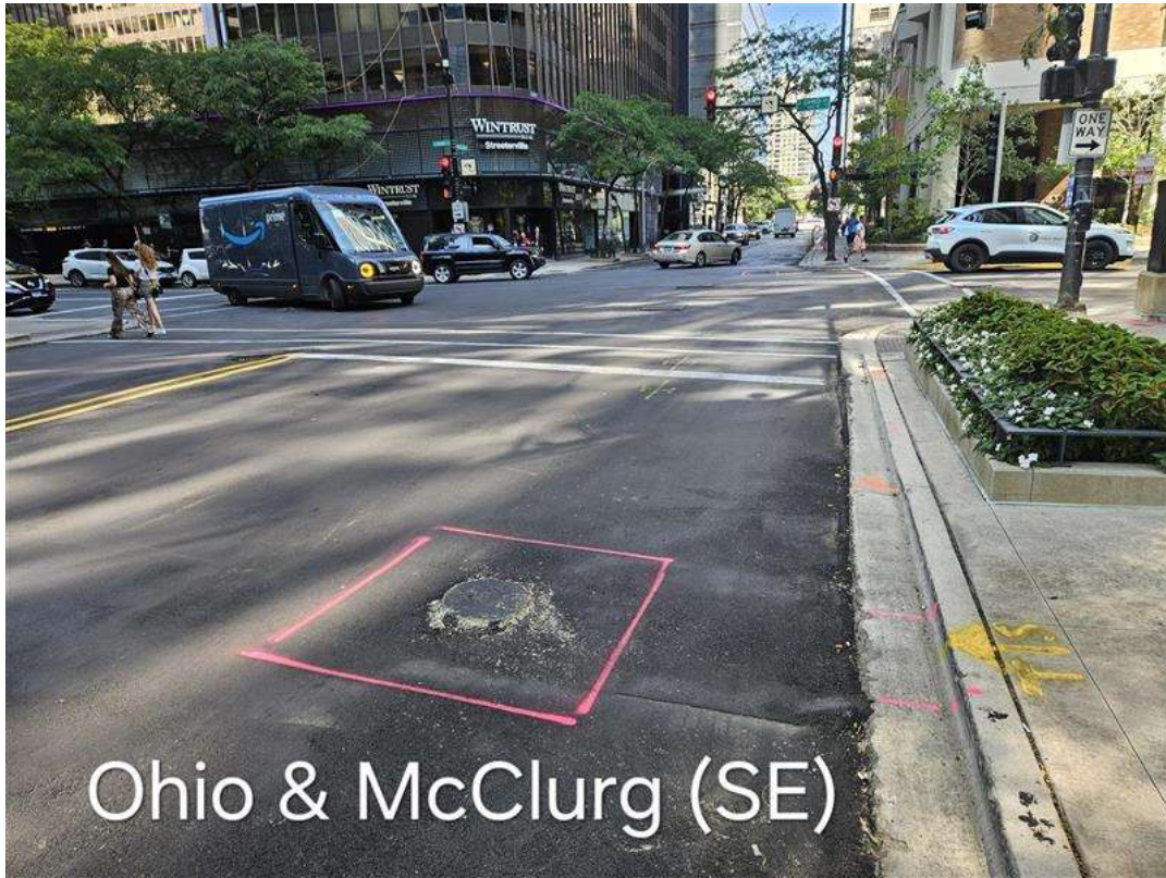
PICTURE 9: DOT1997580 - BEFORE EXCAVATION
