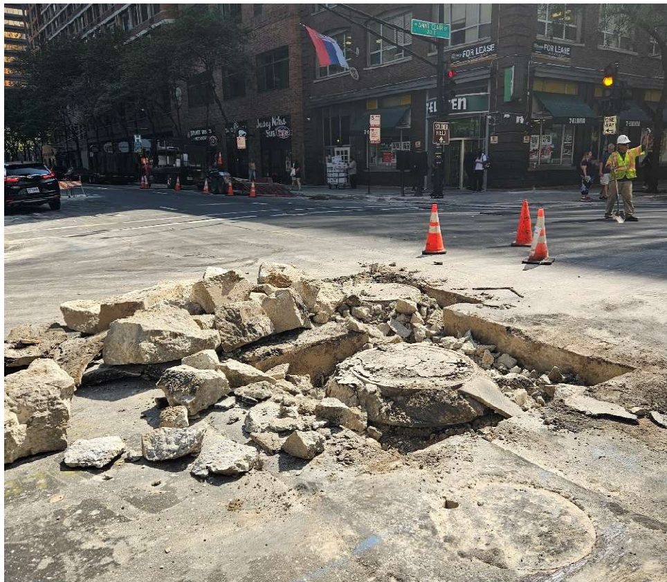
PICTURE 8: DOT1997577 - EXCAVATION 2 & 3 AFTER EXCAVATION
