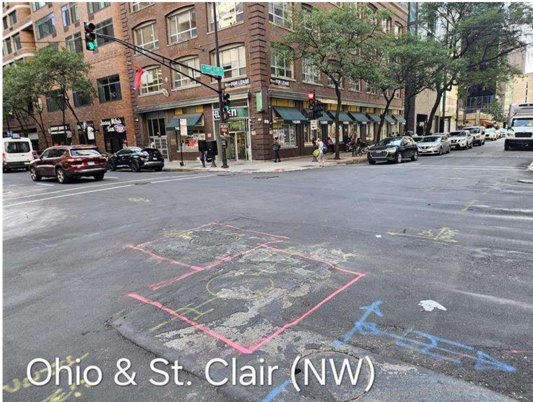
PICTURE 7: DOT1997577 - EXCAVATION 2 & 3 BEFORE EXCAVATION
