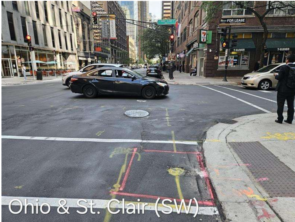
PICTURE 3: DOT1992950 - EXCAVATION 2 BEFORE EXCAVATION
