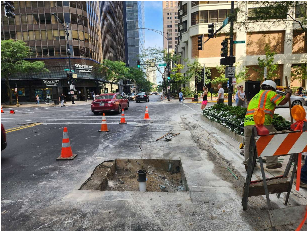
PICTURE 10: DOT1997580 - AFTER EXCAVATION
