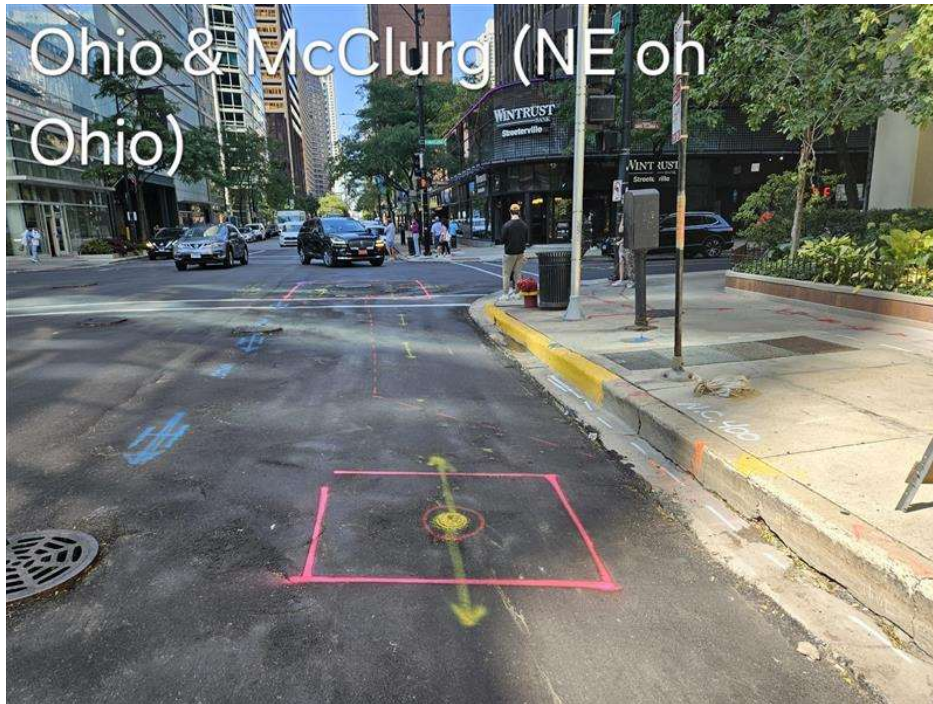
PICTURE 11: DOT1992955 – EXCAVATION 1 BEFORE EXCAVATION
