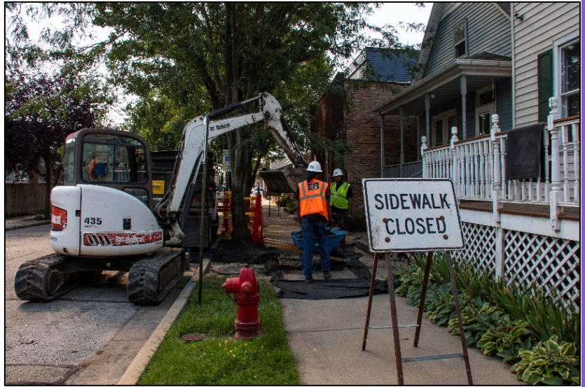
Residential soil excavation as part of EPA's 2018 short-term cleanup.
