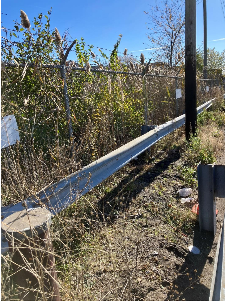
Photograph showing well MW-4S (bottom left corner) and a nearby pole coated in a black substance (right side)
