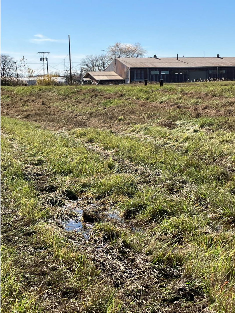
Some ponding observed onsite, but outside of the landfill and sediment caps
