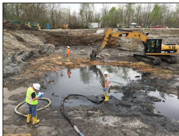
Excavation at NPL-4; the water was pumped into a holding tank, characterized for hazardous waste and disposed of properly. Source:
