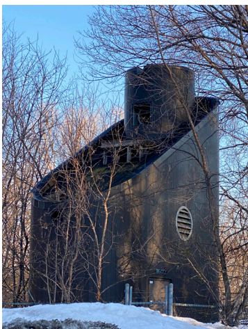
Building that housed the pump and treat system on the General Mills site.
