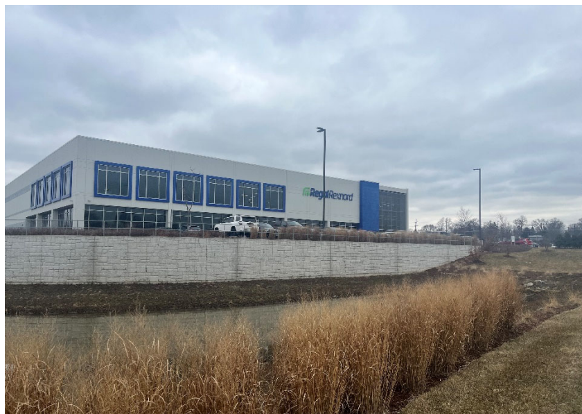
The Rexnord property along Curtiss Street. An AS/SVE system was installed to address the vapor intrusion concerns at the property.
