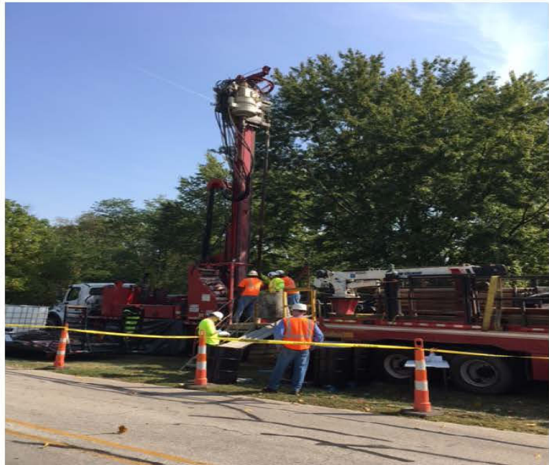
A contractor collecting groundwater samples.
