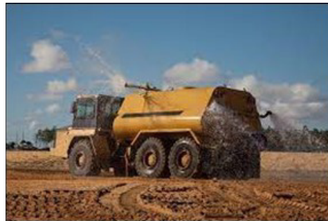
1: Example of water tanker wetting soil to prevent airborne dust.
