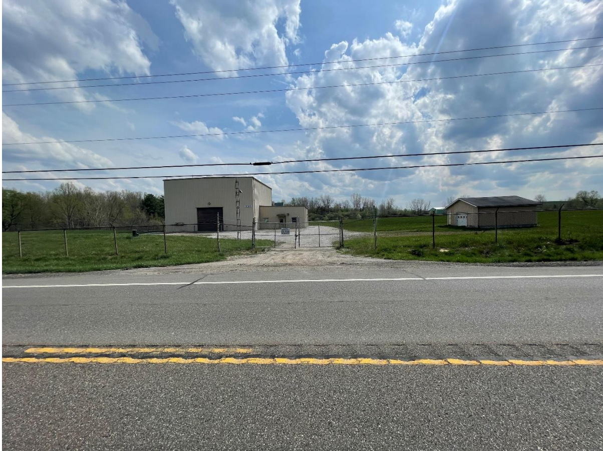
Photo 1: Site entrance gate.
