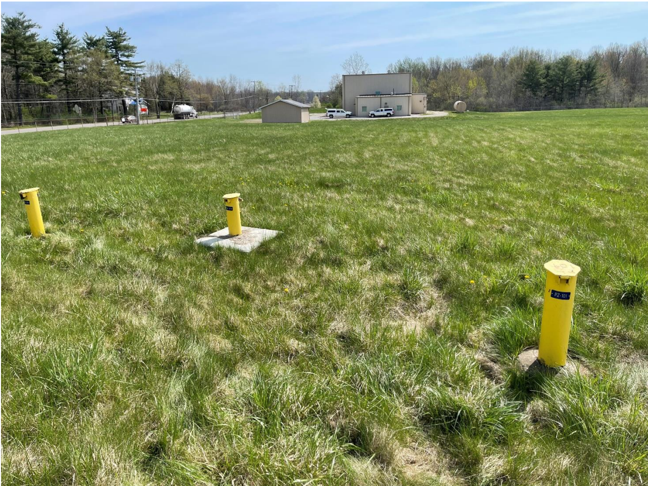
Photo 3: Monitoring well cluster.
