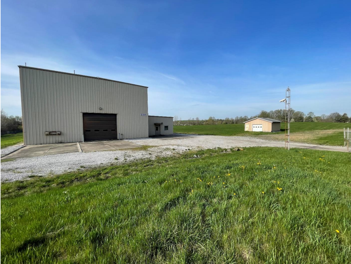
Photo 2: Former water treatment system building.
