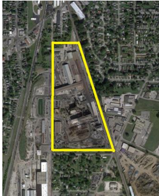
Nucor Steel Marion, Inc. facility in Marion, Ohio
