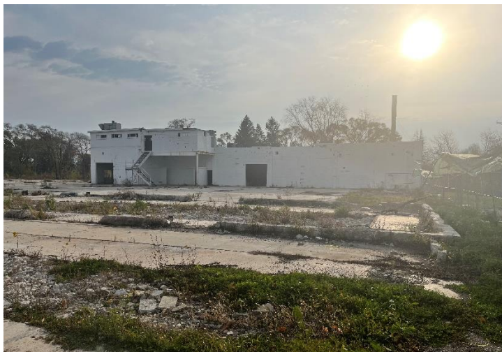
View northeast of grassy and paved areas surrounding the Amcast North building.
