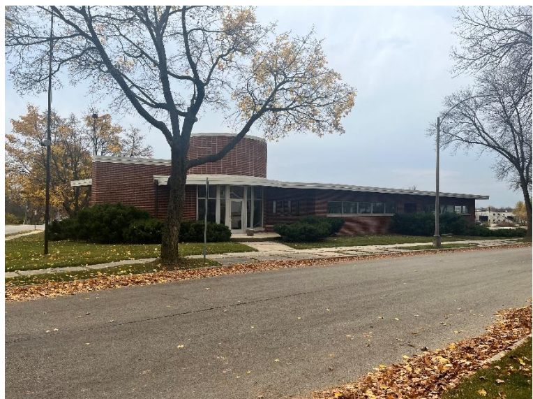
View southeast of Amcast South showing the office building.
