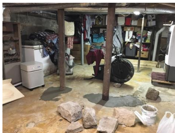
Figure 9-3. Holes in Floor Sealed with Hydraulic Cement
