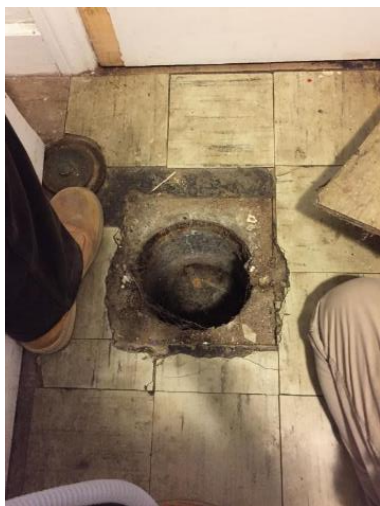
Figure 9-4. Dry Sump Prior to Filling with Concrete
