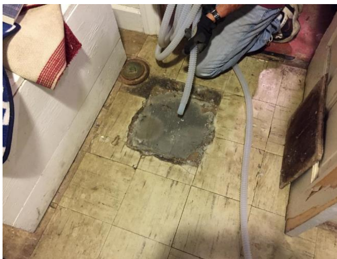
Figure 9-5. Dry Sump After Filling with Concrete
