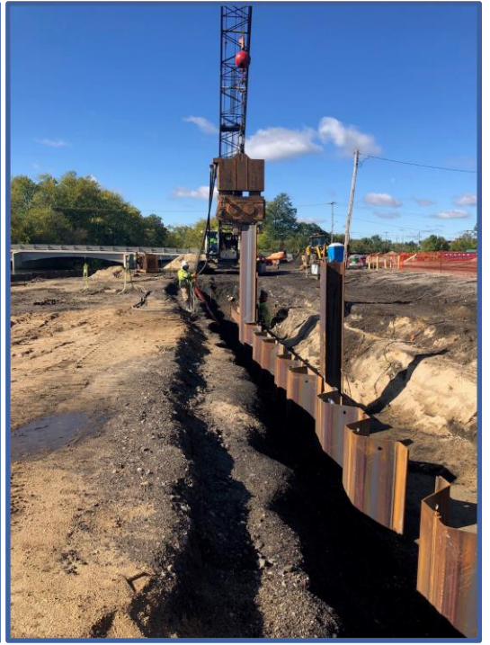
Example of metal sheet piling installation.
