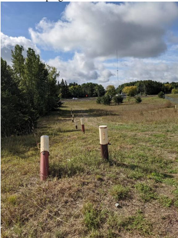
Figure D-10: View south to the Phase II (upgradient) air sparge line, showing a directionally-drilled air sparge well head.
