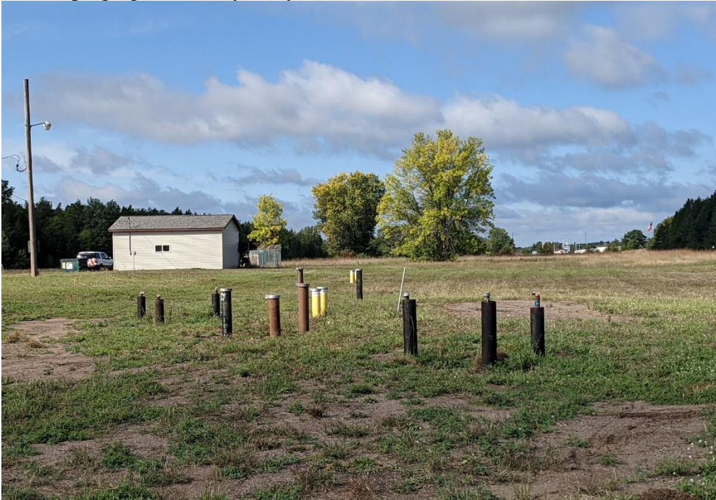
Figure D-13: Biosparge well nests AI-92 (AI-92A/B/C) and AI-94 (AI-94A/B/C) and observation well nests AI-93 (AI-93A/B/C) and AI-95 (AI-95B/C), constructed for Phase 1 of the biosparging treatability study.
