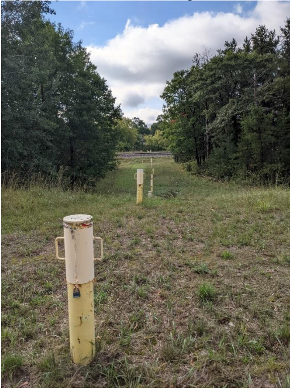
Figure D-10: View south to the Phase II (upgradient) air sparge line, showing a directionally-drilled air sparge well head.
