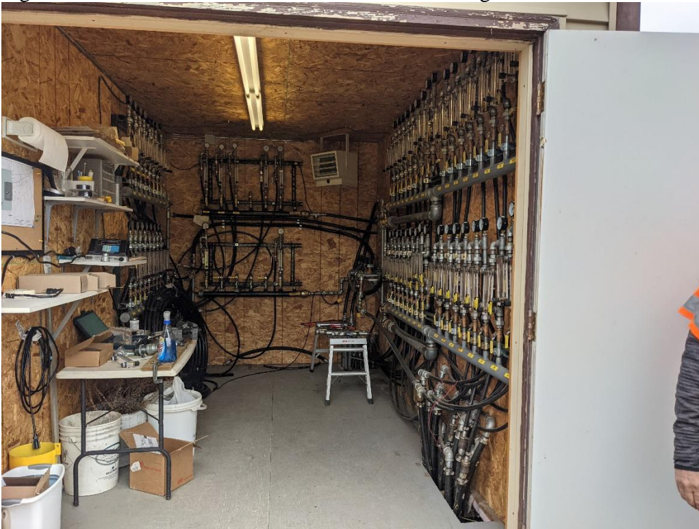
Figure D-4: Air distribution manifold.
