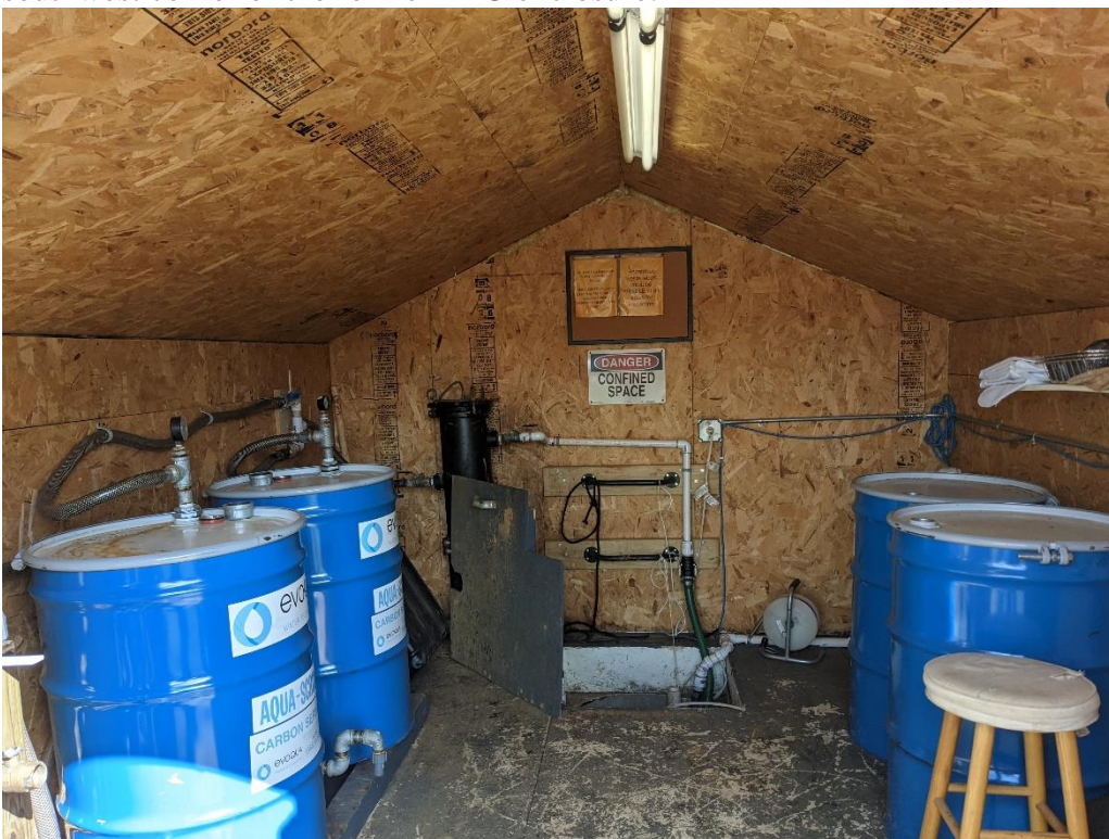
Figure D-12: Activated carbon treatment system in the leachate treatment building at the southwest corner of the former LTU enclosure.
