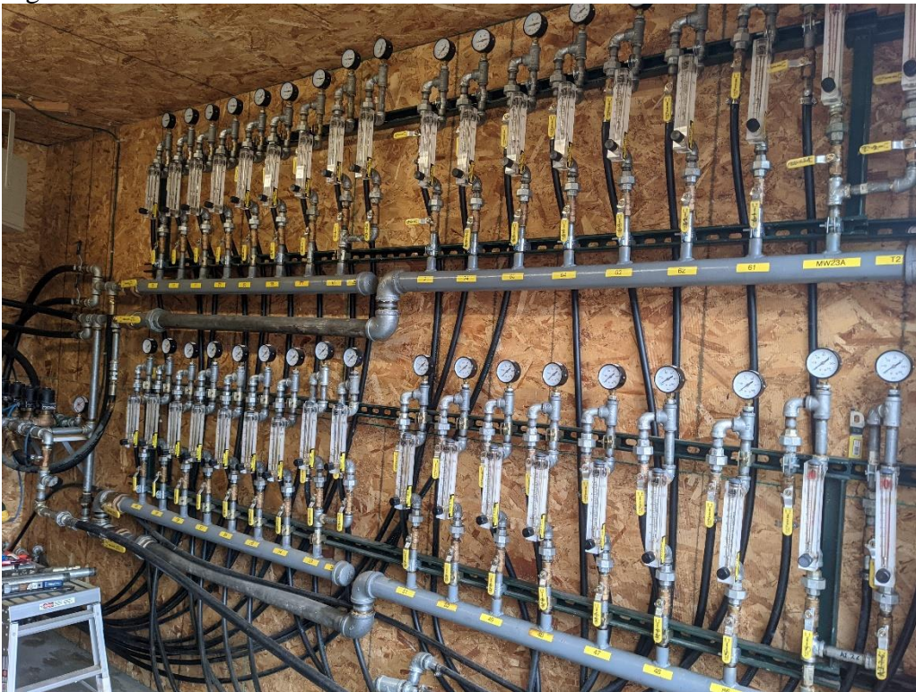
Figure D-4: Air distribution manifold.
