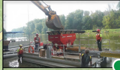
SMA 2-5 - Armor stone placement at the perimeter of a CCS cap
