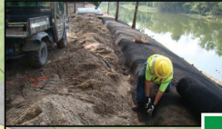
BMA 2-3 - Bank stabilization and canopy management
