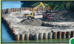
SMA 2-3 - Sediment removal
