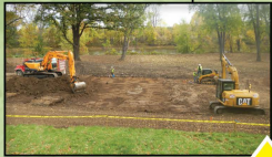
Floodplain - Soil removal and replacement
