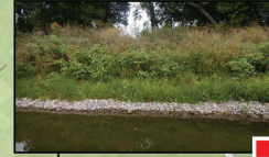
BMA 4-6 - Bank stabilization
