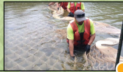
SMA 3-2 - CCS capping (Cellular Containment System)
