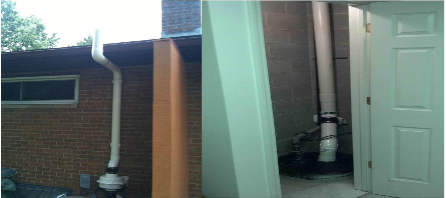
FIGURE 12: SSD System Installation—Exterior and Exterior Components
