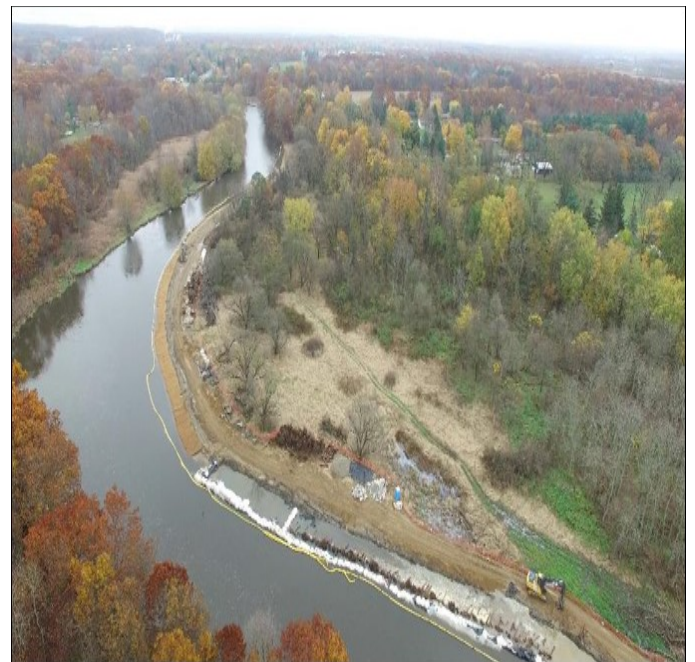
Bank work in Area 3.
