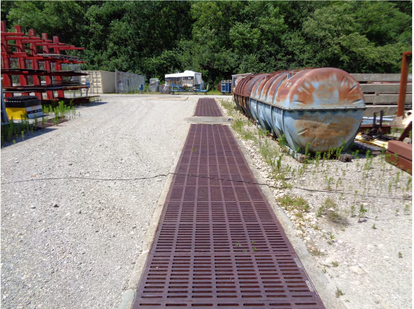
Photograph # 1 Inlet Sump Pump Grating
