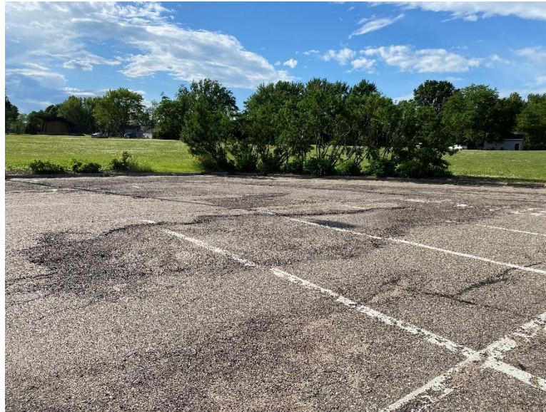
6/11/2020: View of City-owned parking lot from the north end of the westernmost row, to the south and northwest. Some asphalt erosion and cracking present.
