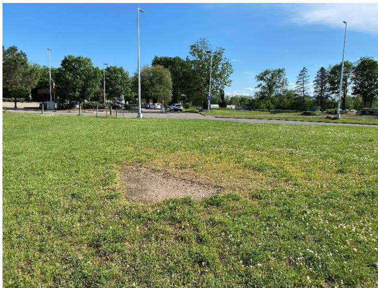
6/11/2020: Grassy cap, view to east and to south. Grass is in good condition over most of the cap, some patchy areas. No cracking, sinking or mounding observed.
