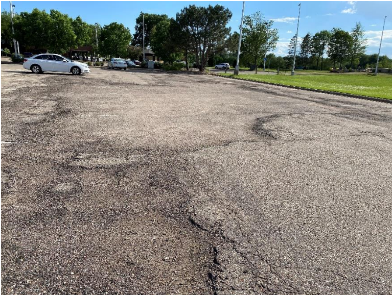
6/11/2020: View of City-owned parking lot from the north end of the westernmost row, to the south and northwest. Some asphalt erosion and cracking present.
