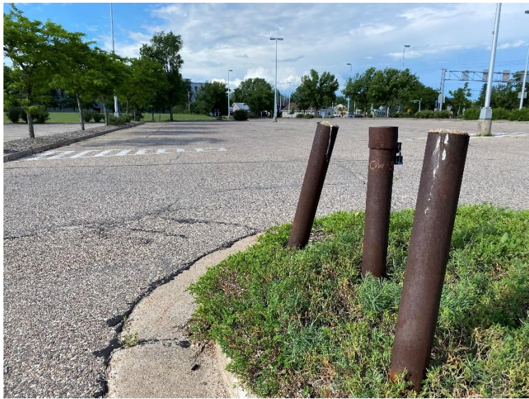
6/11/2020: View of OW08 (from south) and OW07A & PZ07B (from east). Monitor wells and bollards are in good condition and secure.
