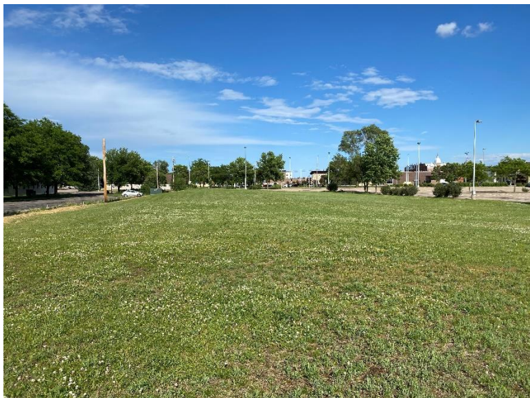
6/11/2020: Grassy cap, view to east and to south. Grass is in good condition over most of the cap, some patchy areas. No cracking, sinking or mounding observed.
