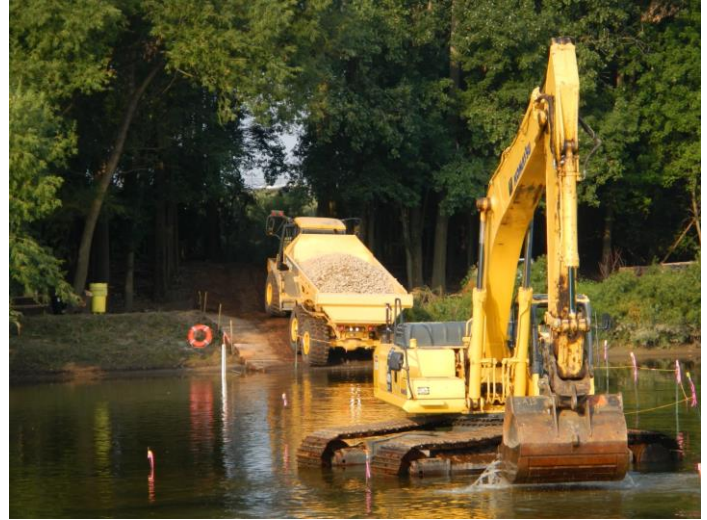
Cap materials being placed in the Tittabawassee River (not from a barge)
