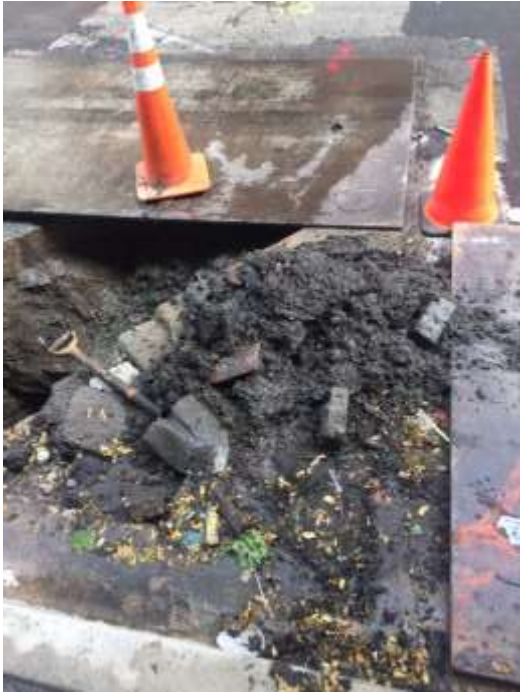
Excavation #1 – Hand Dig
