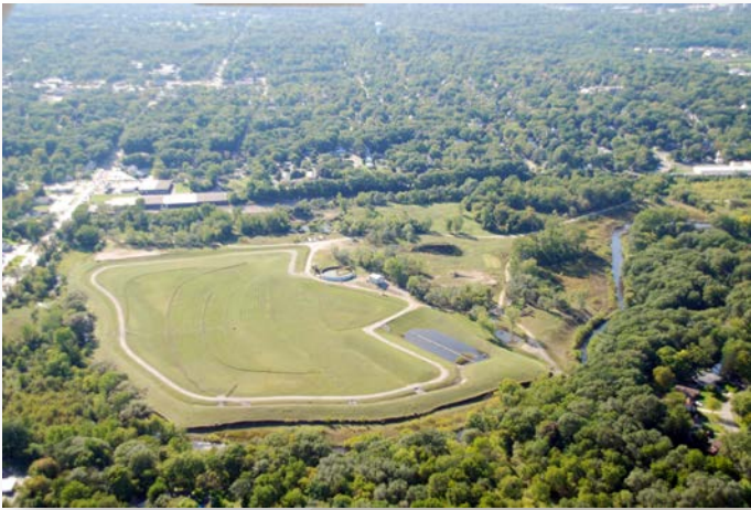
Aerial photo of Allied Landfill and Portage Creek.
